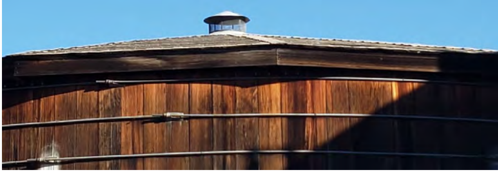
Close up #2 of redwood tank roof, showing small superstructure for ventilation and shingles, taken 11/10/22, Photo #135453, from Photolog BS-01.
