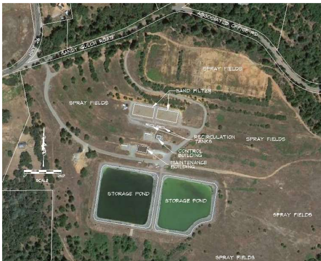
Figure 2: West Point Wastewater Treatment Facility
