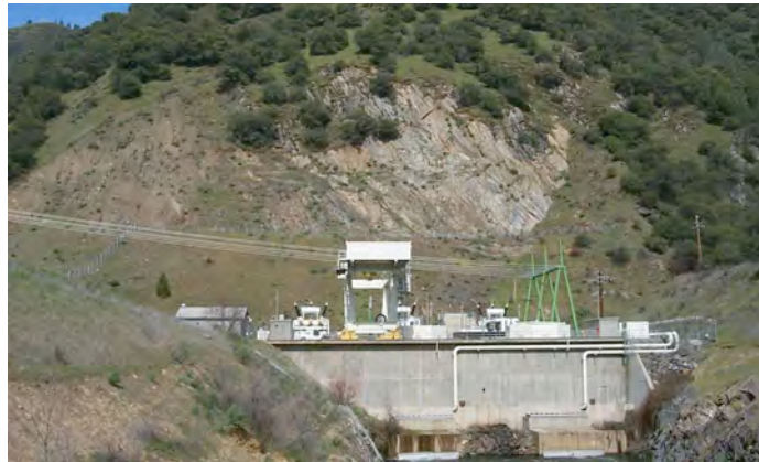
Collierville Powerhouse at Clarks Flat on North Fork Stanislaus
