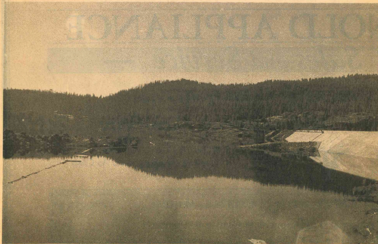
THE NEW SPICER MEADOW dam and reservoir will provide the Central Sierras with a new recreation area. Although the reservoir is closed to the public currently, due to logging operations and the construction of recreation facilities, it is expected to open next summer with a boat launch, picnic and campground sites.
