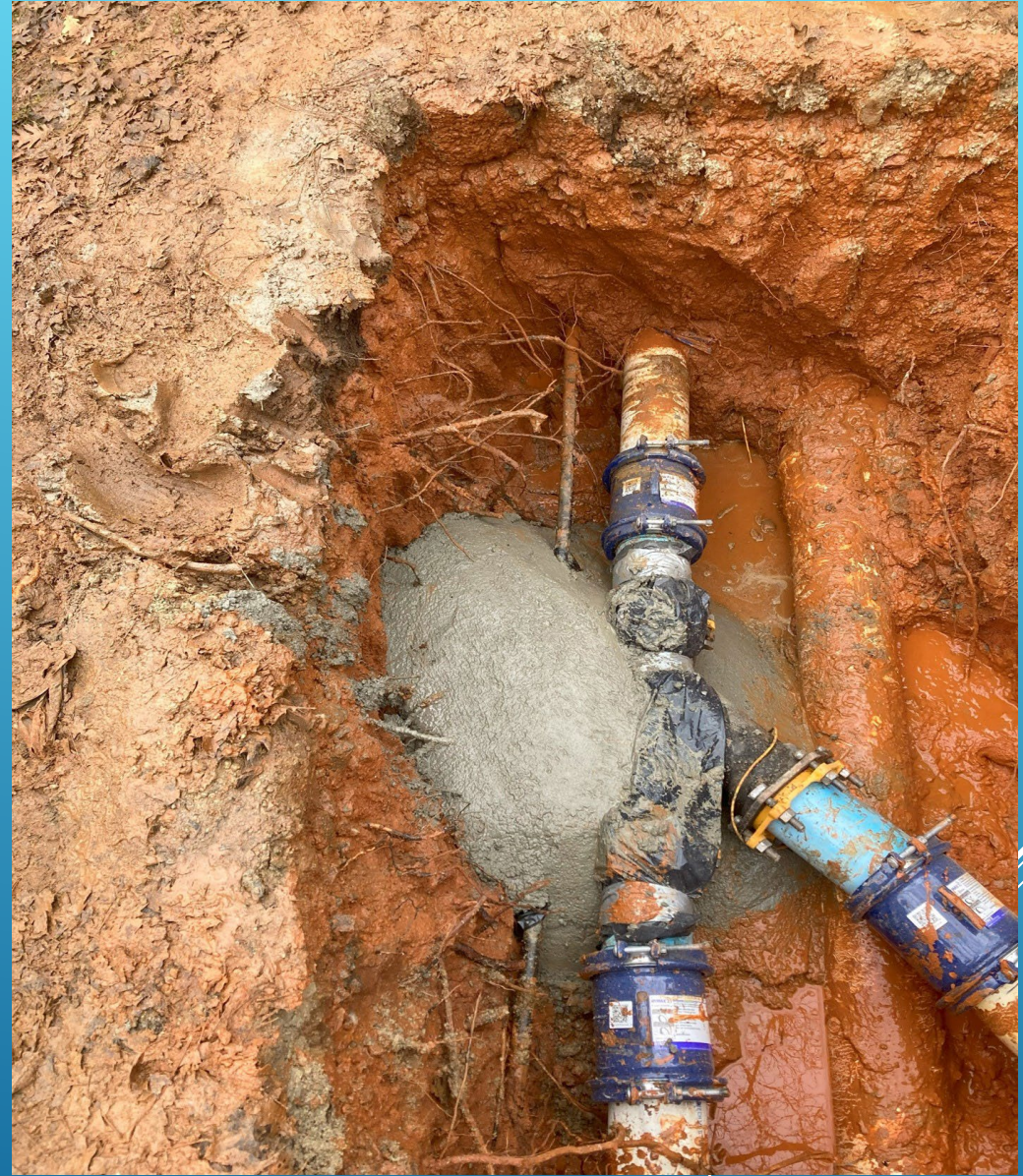
4-INCH BY 6-INCH WYE REPLACEMENT – MIDDLE FORK RAW LINE – WEST POINT
