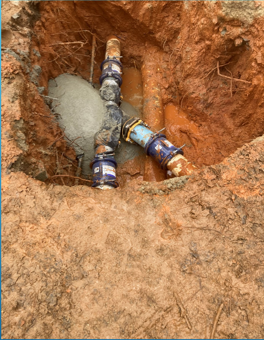
4-INCH BY 6-INCH WYE REPLACEMENT – MIDDLE FORK RAW LINE – WEST POINT
