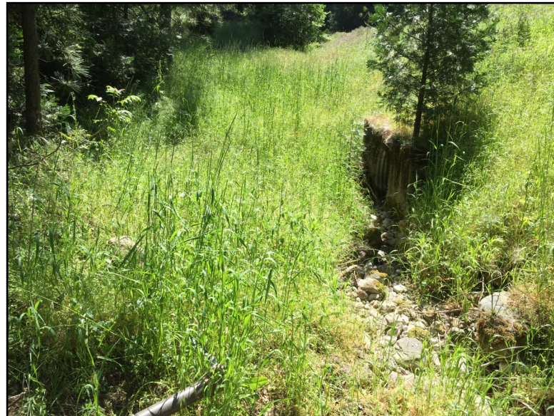
Photo 6. Ditch south of Red Apple Drive, facing west. May 25, 2017.
