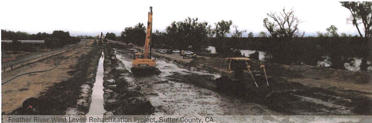
Feather River West Levee Rehabilitation Project, Sutter County, CA
