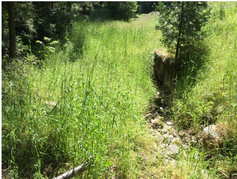
Photo 5. View of ephemeral drainage ED-2, facing west. Photo taken on May 25, 2017.
