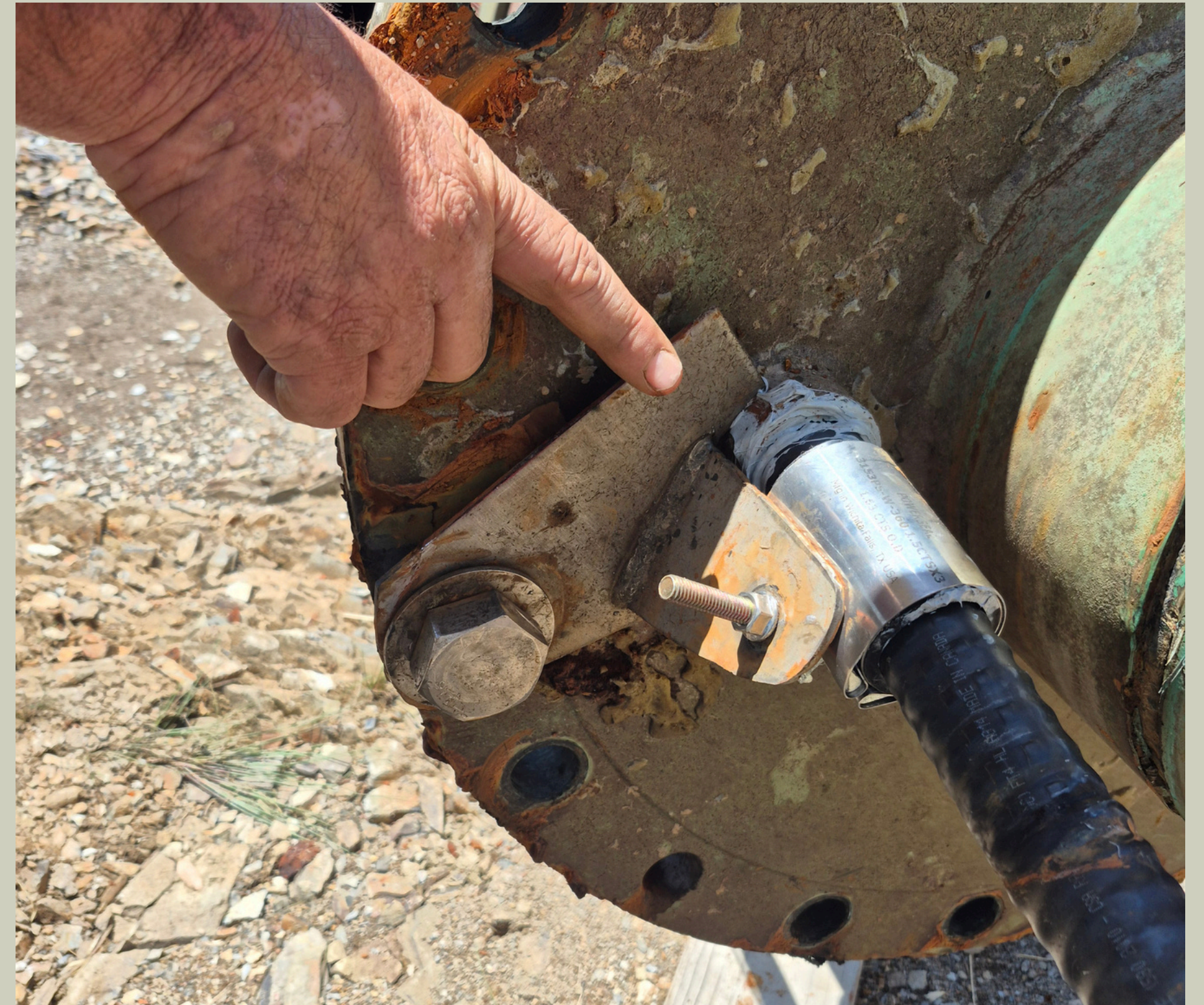
Copper Cove - RWPS - Pump Replacement Project
