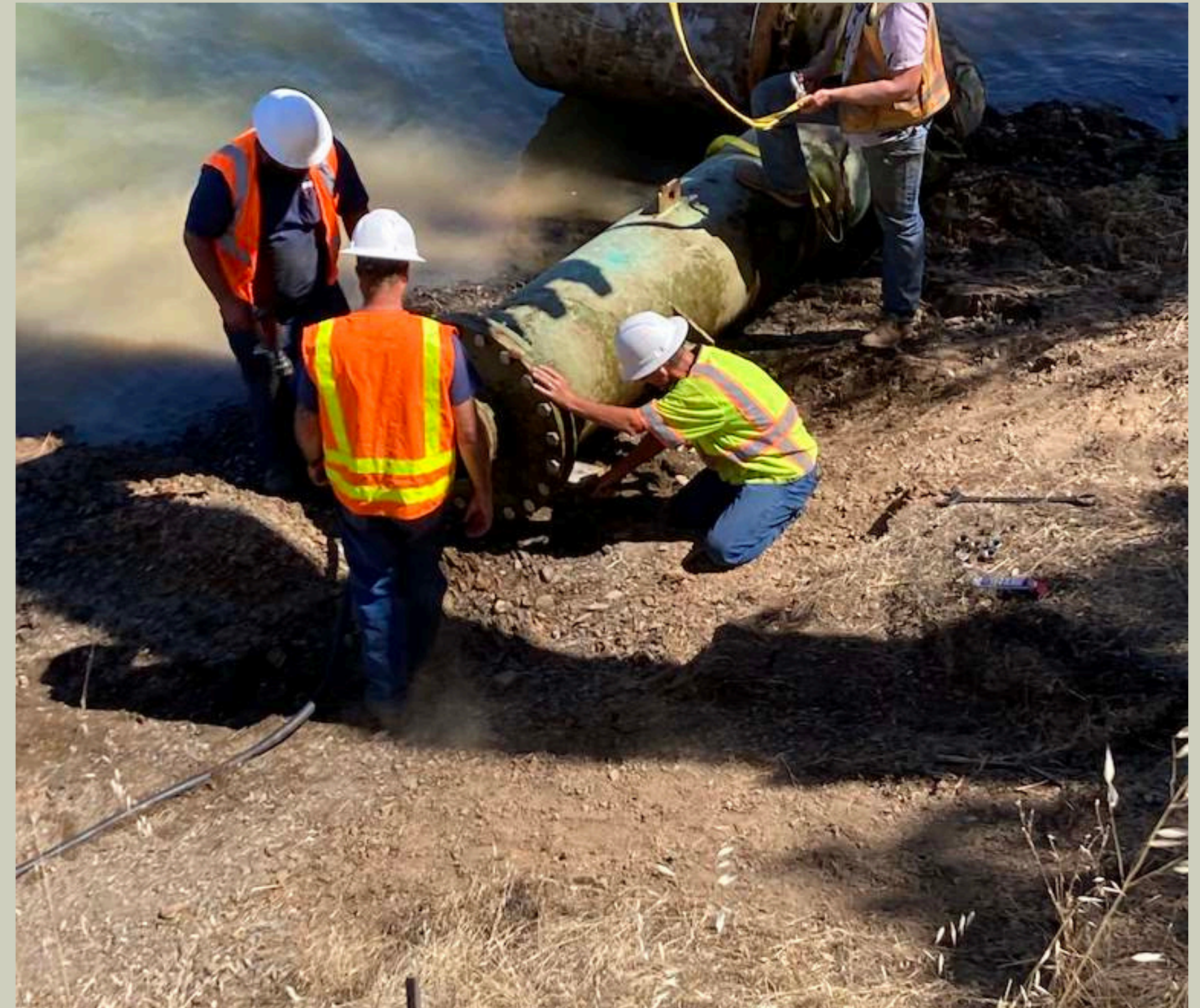
Copper Cove - RWPS - Pump Replacement Project
