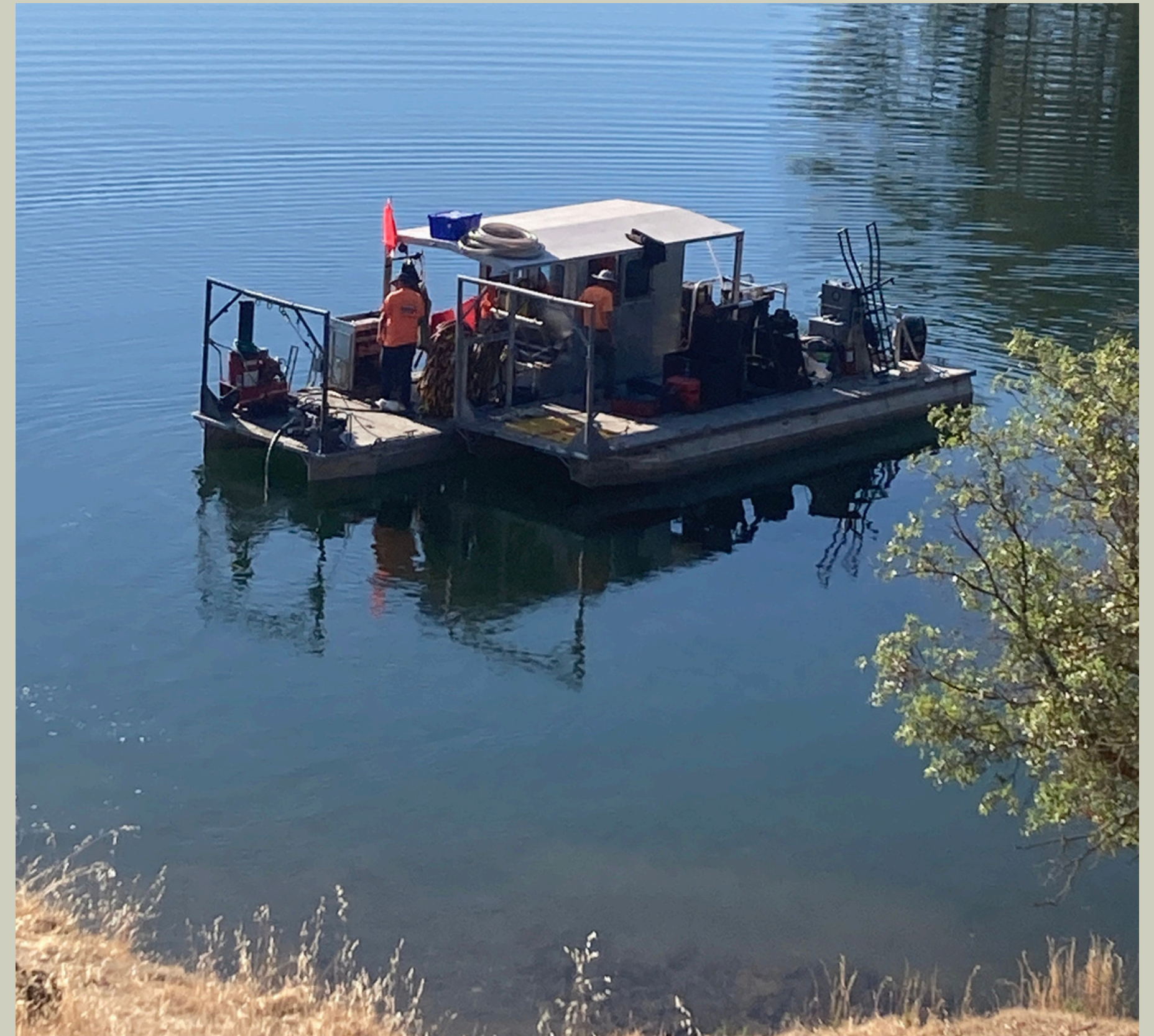
Copper Cove - RWPS - Pump Replacement Project
