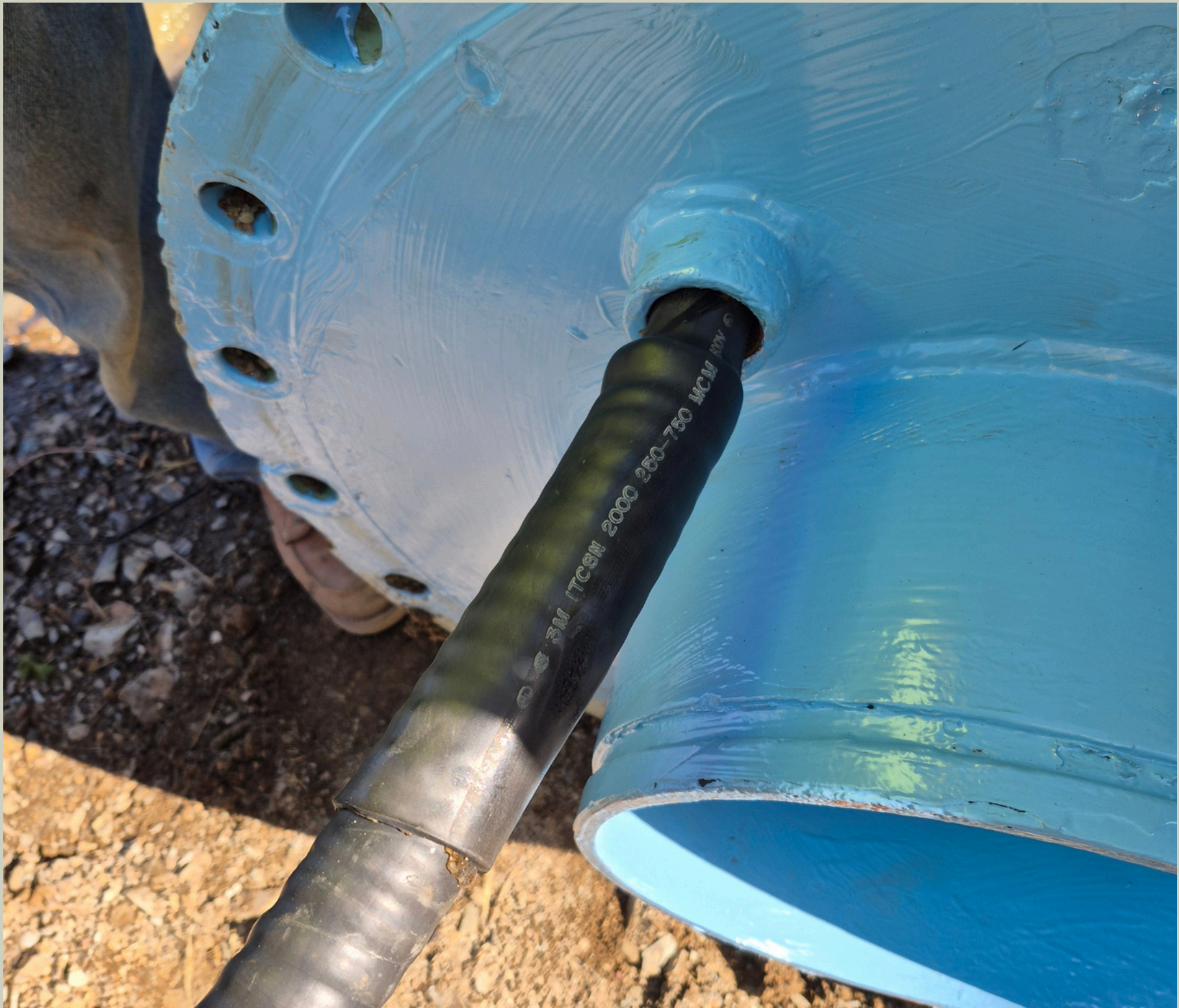
Copper Cove - RWPS - Pump Replacement Project
