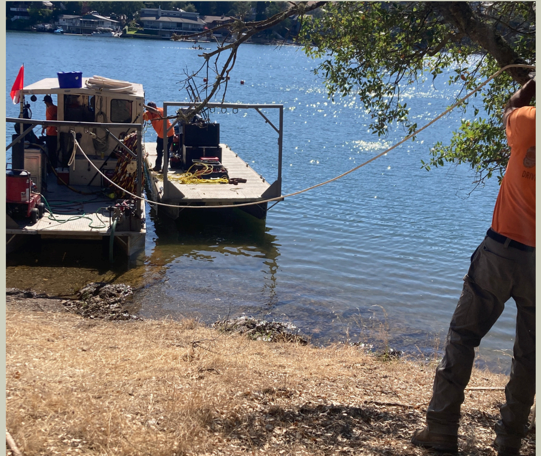
Copper Cove - RWPS - Pump Replacement Project
