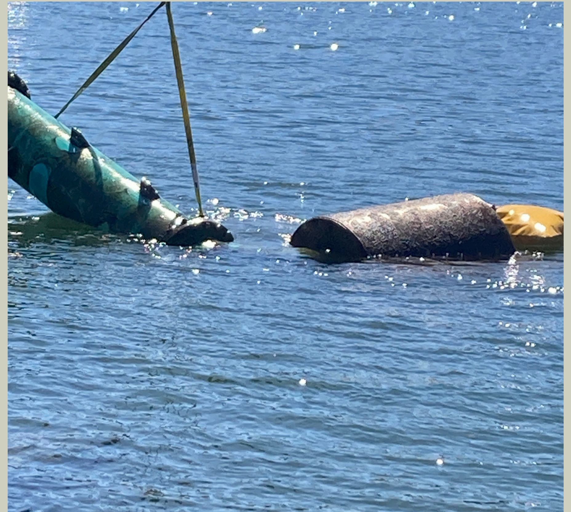
Copper Cove - RWPS - Pump Replacement Project
