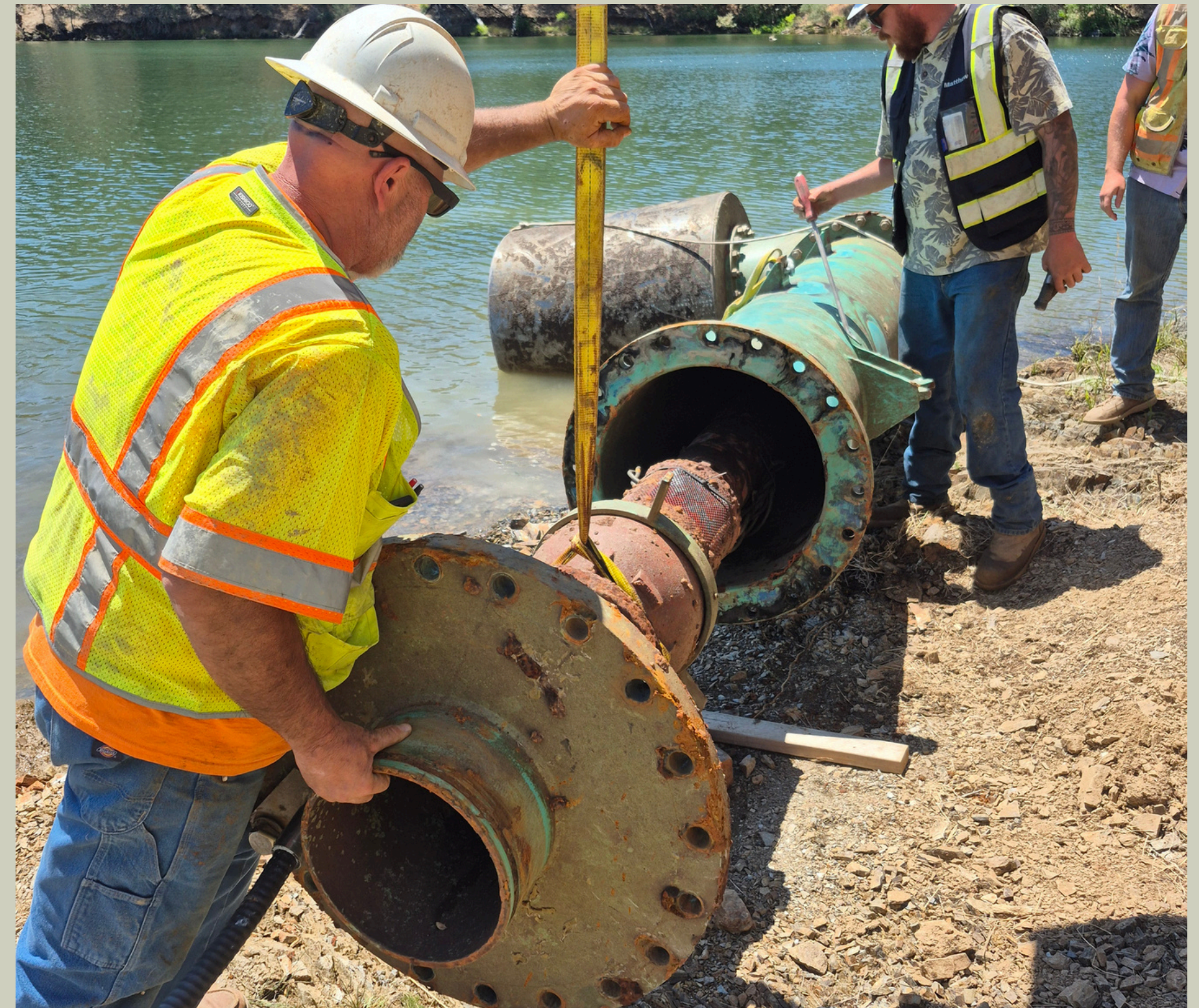
Copper Cove - RWPS - Pump Replacement Project
