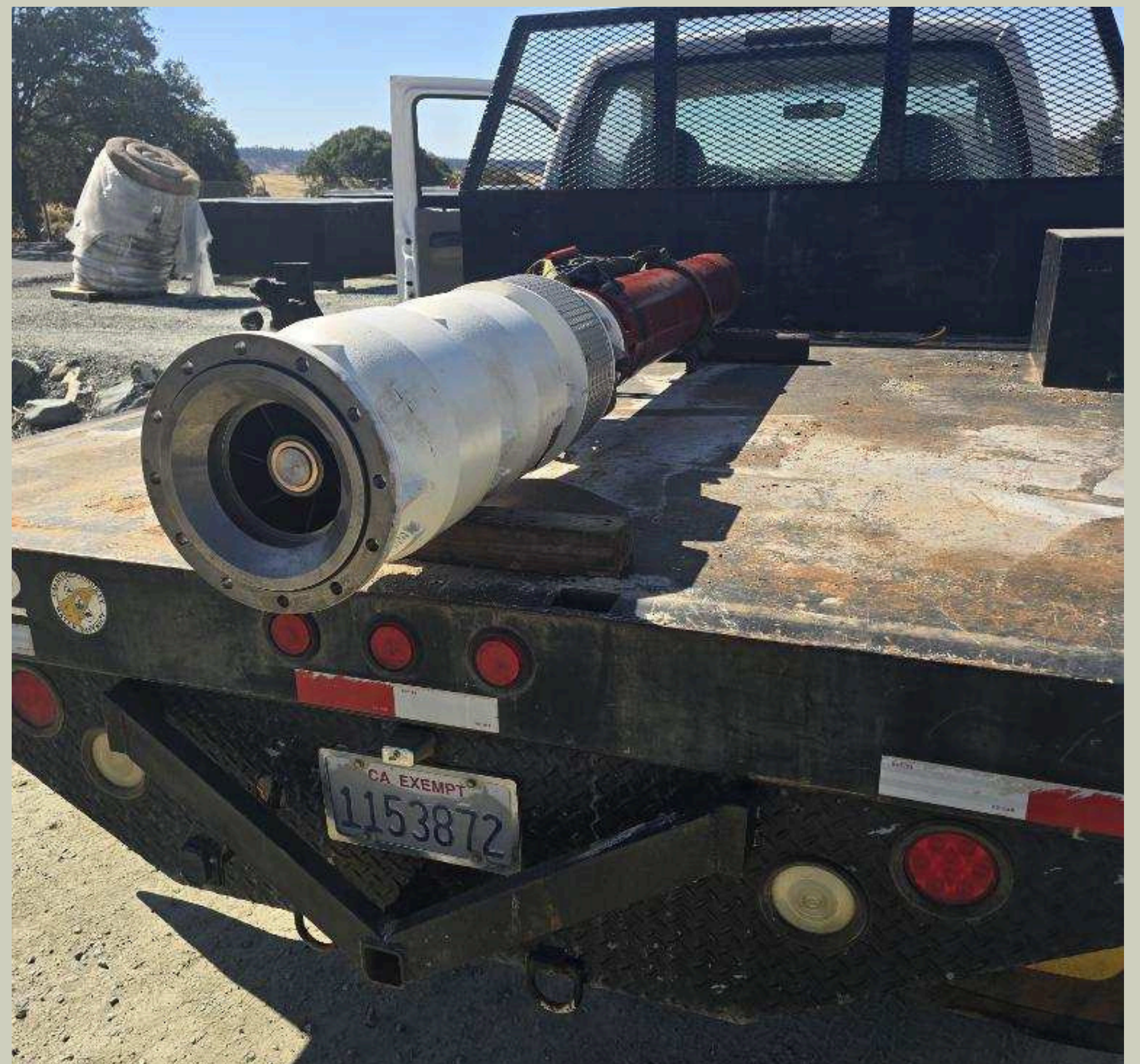
Copper Cove - RWPS - Pump Replacement Project
