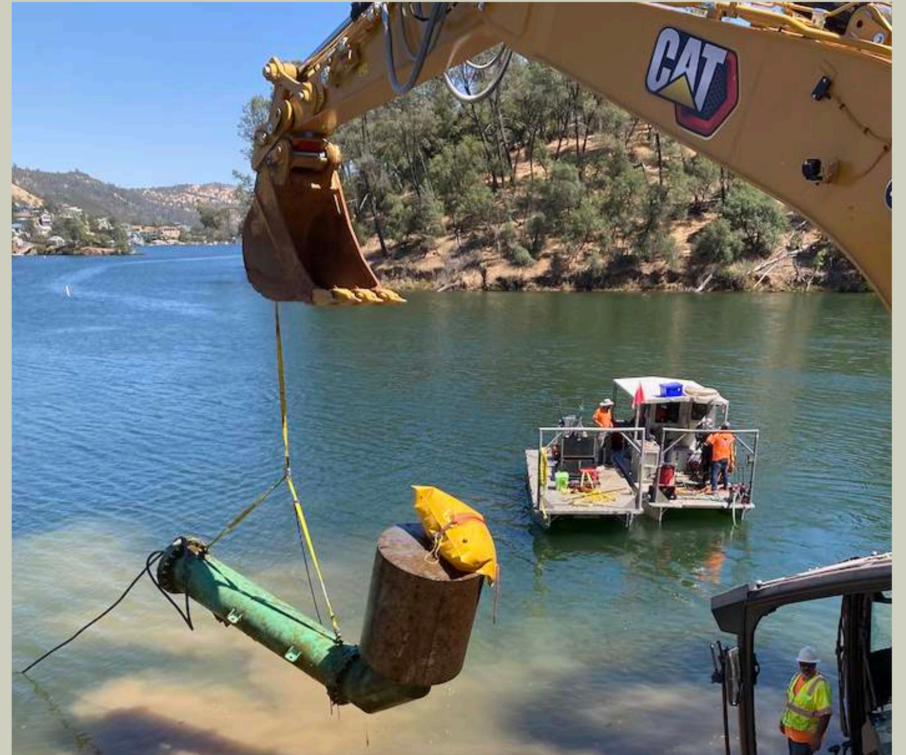
Copper Cove - RWPS - Pump Replacement Project
