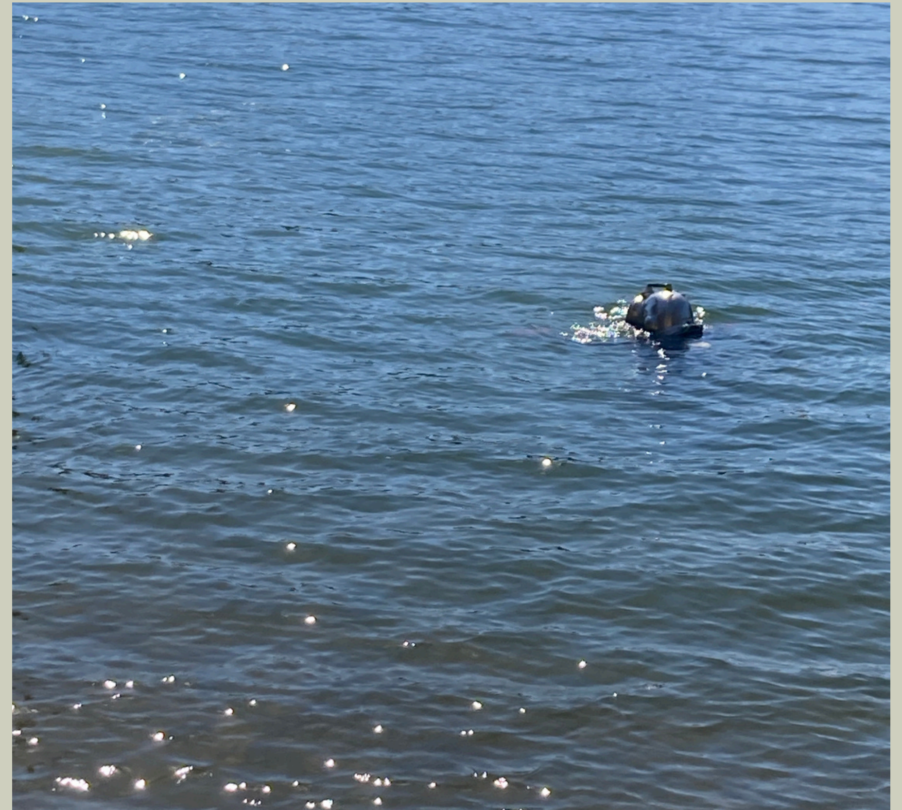
Copper Cove - RWPS - Pump Replacement Project
