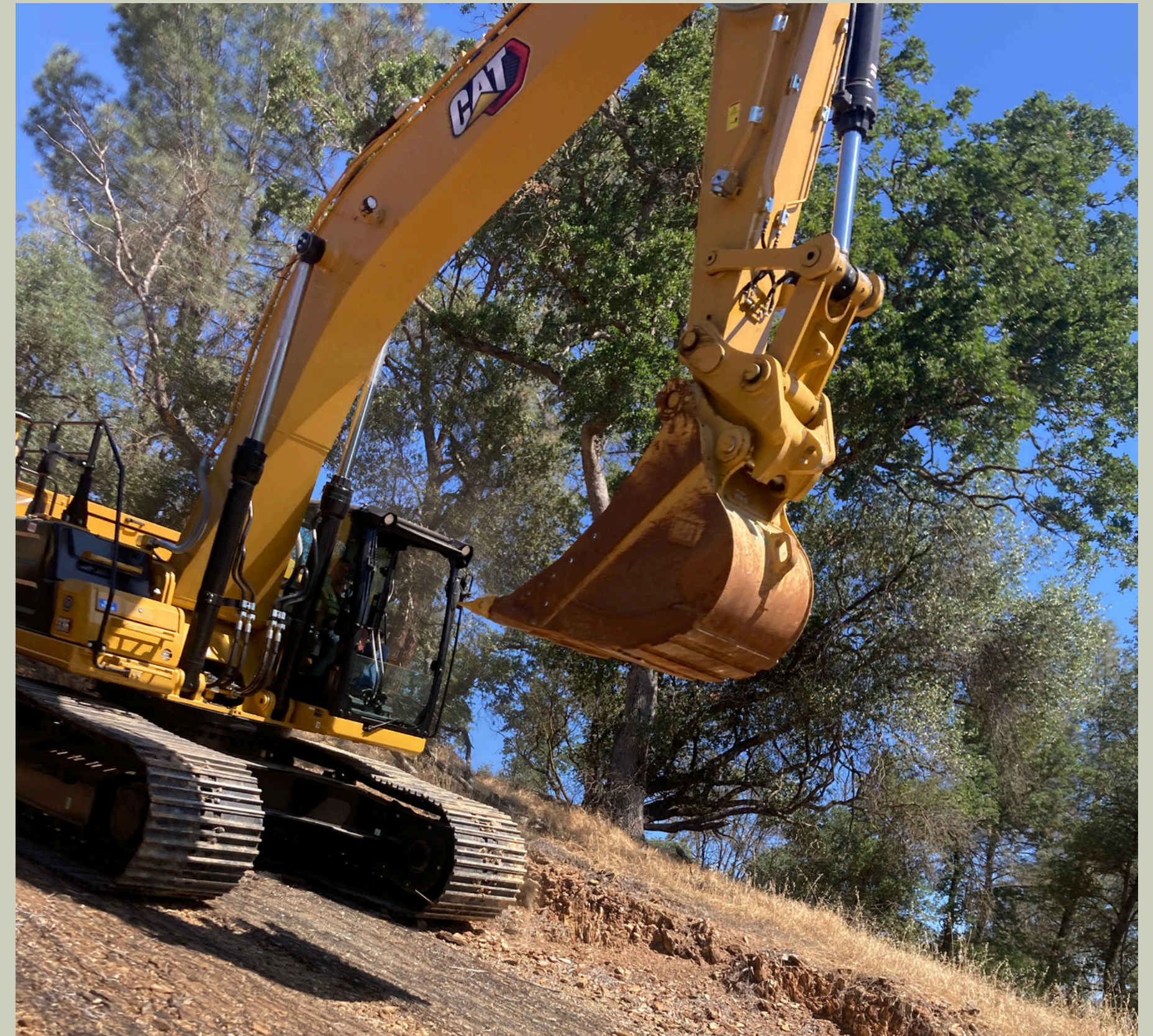
Copper Cove - RWPS - Pump Replacement Project
