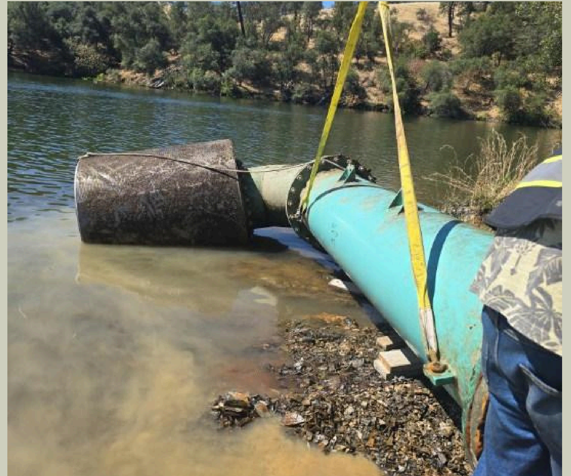
Copper Cove - RWPS - Pump Replacement Project
