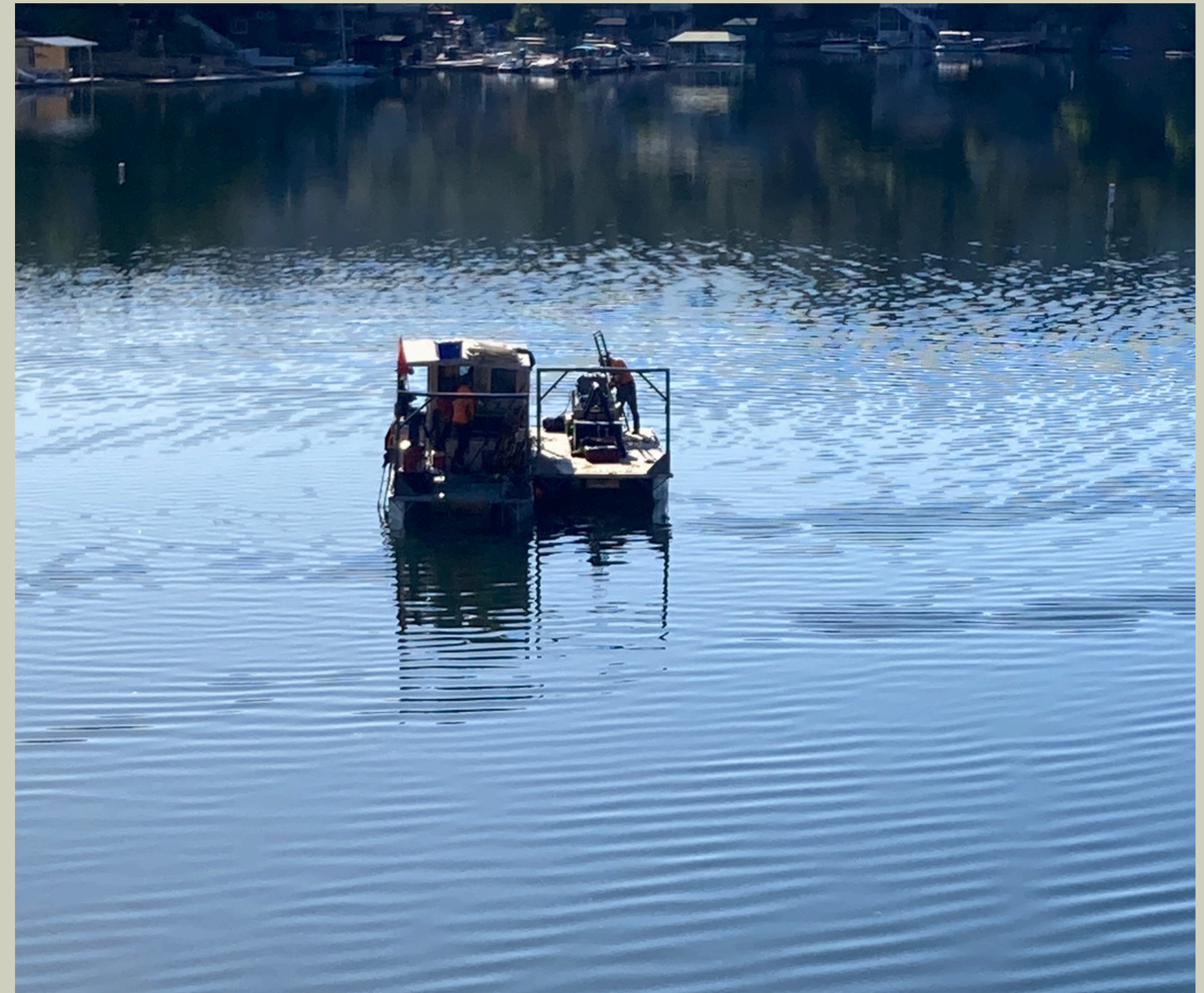
Copper Cove - RWPS - Pump Replacement Project
