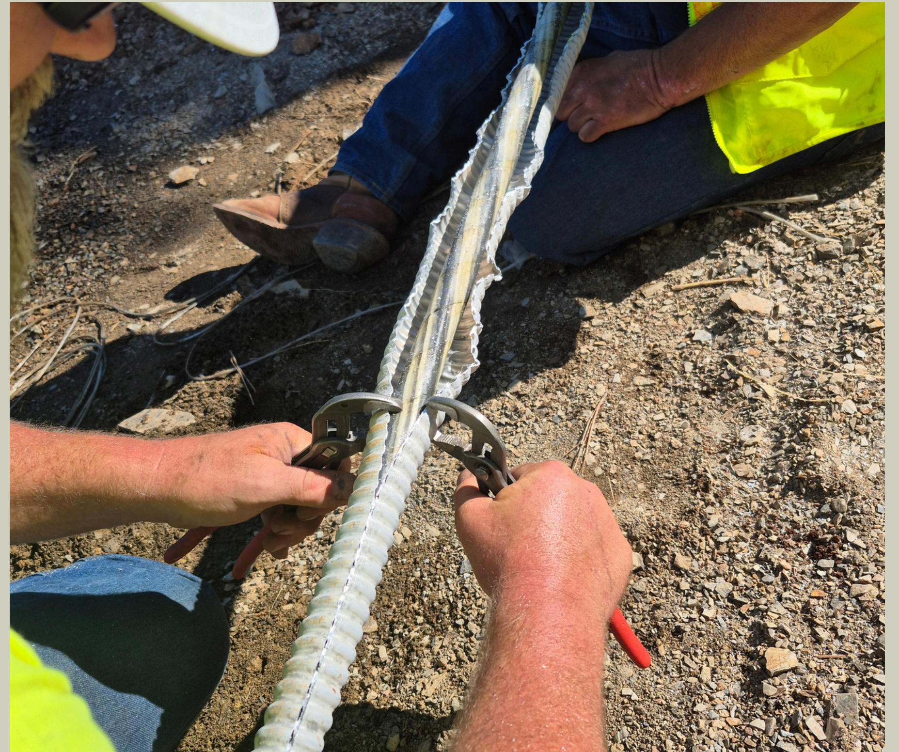
Copper Cove - RWPS - Pump Replacement Project
