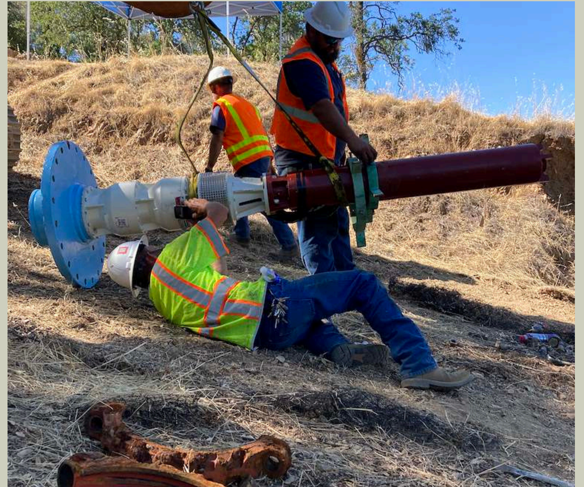
Copper Cove - RWPS - Pump Replacement Project
