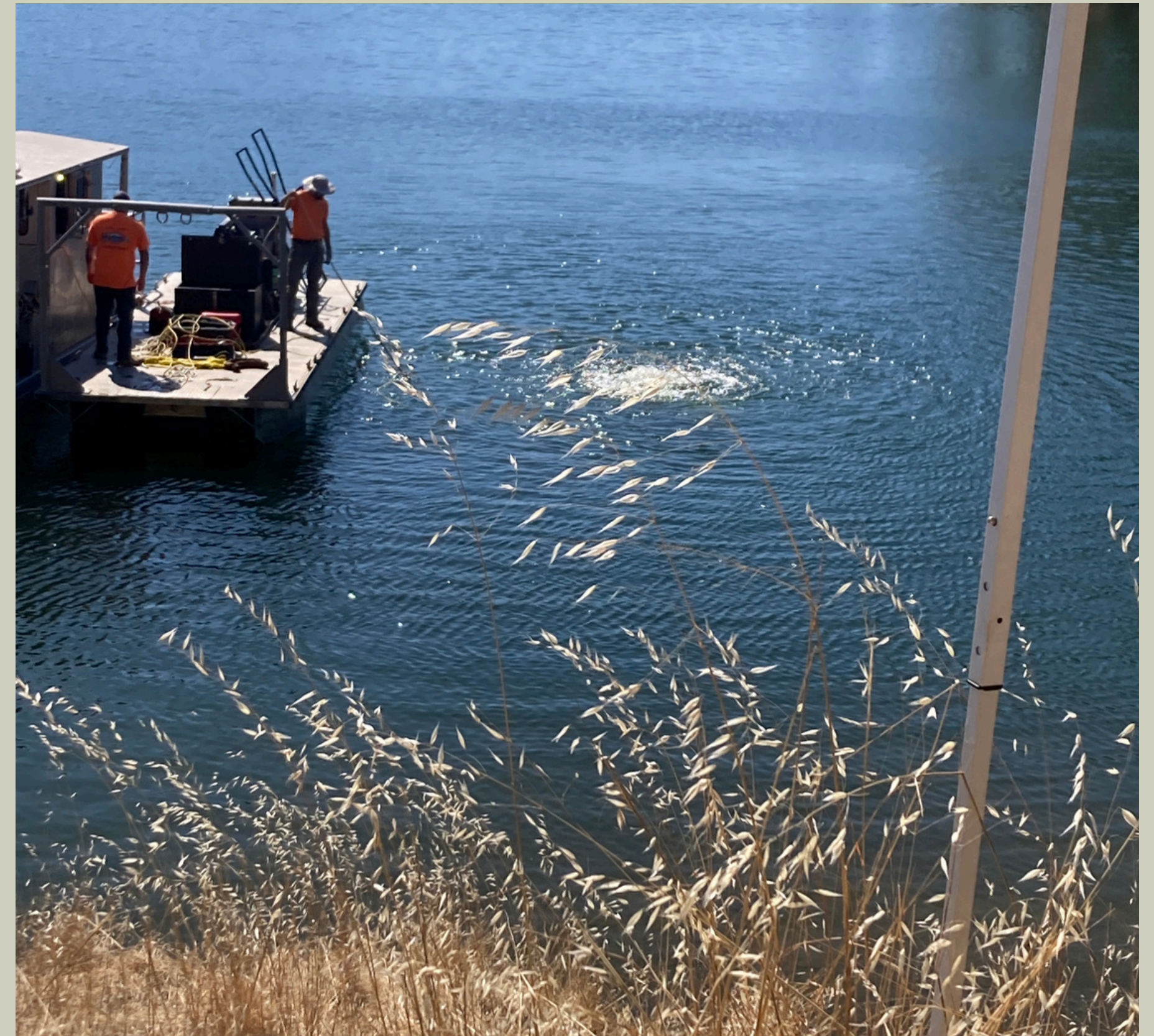
Copper Cove - RWPS - Pump Replacement Project
