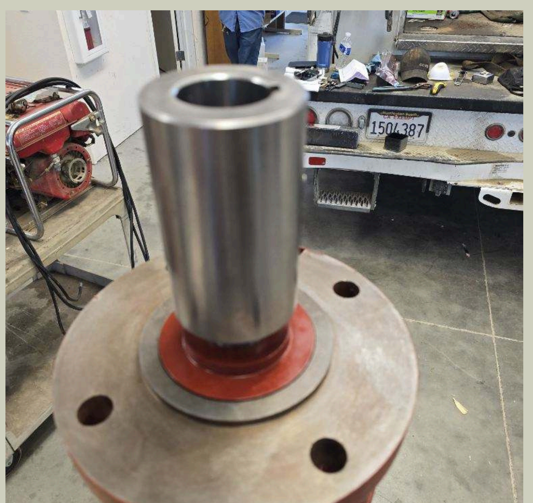
Copper Cove - RWPS - Pump Replacement Project
