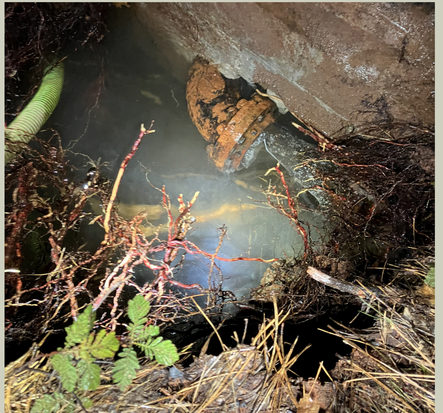
Leak at PRV 30 on Thunderbolt - Ebbetts Pass
