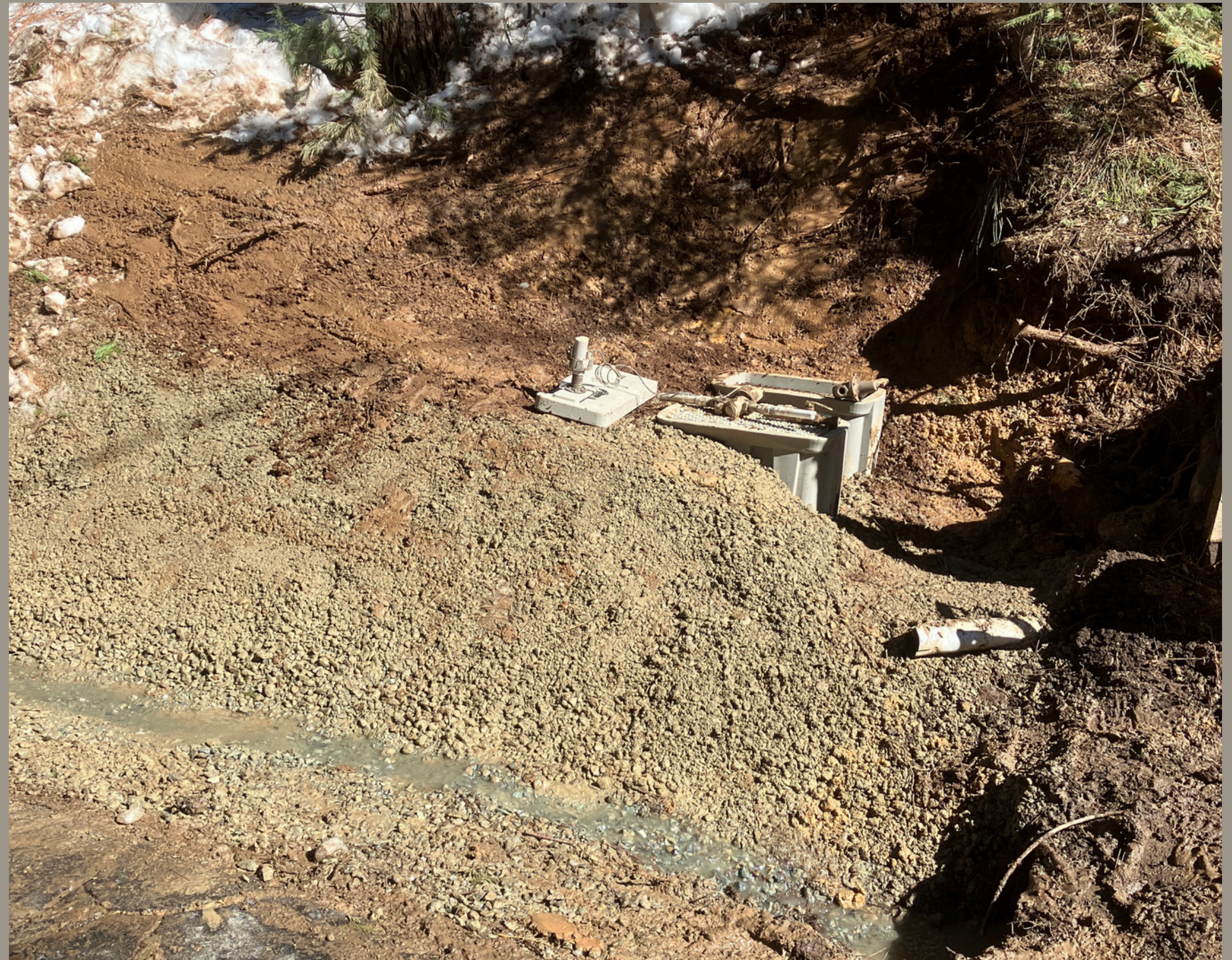
Lilac Drive Service Line Repair - Ebbetts Pass
