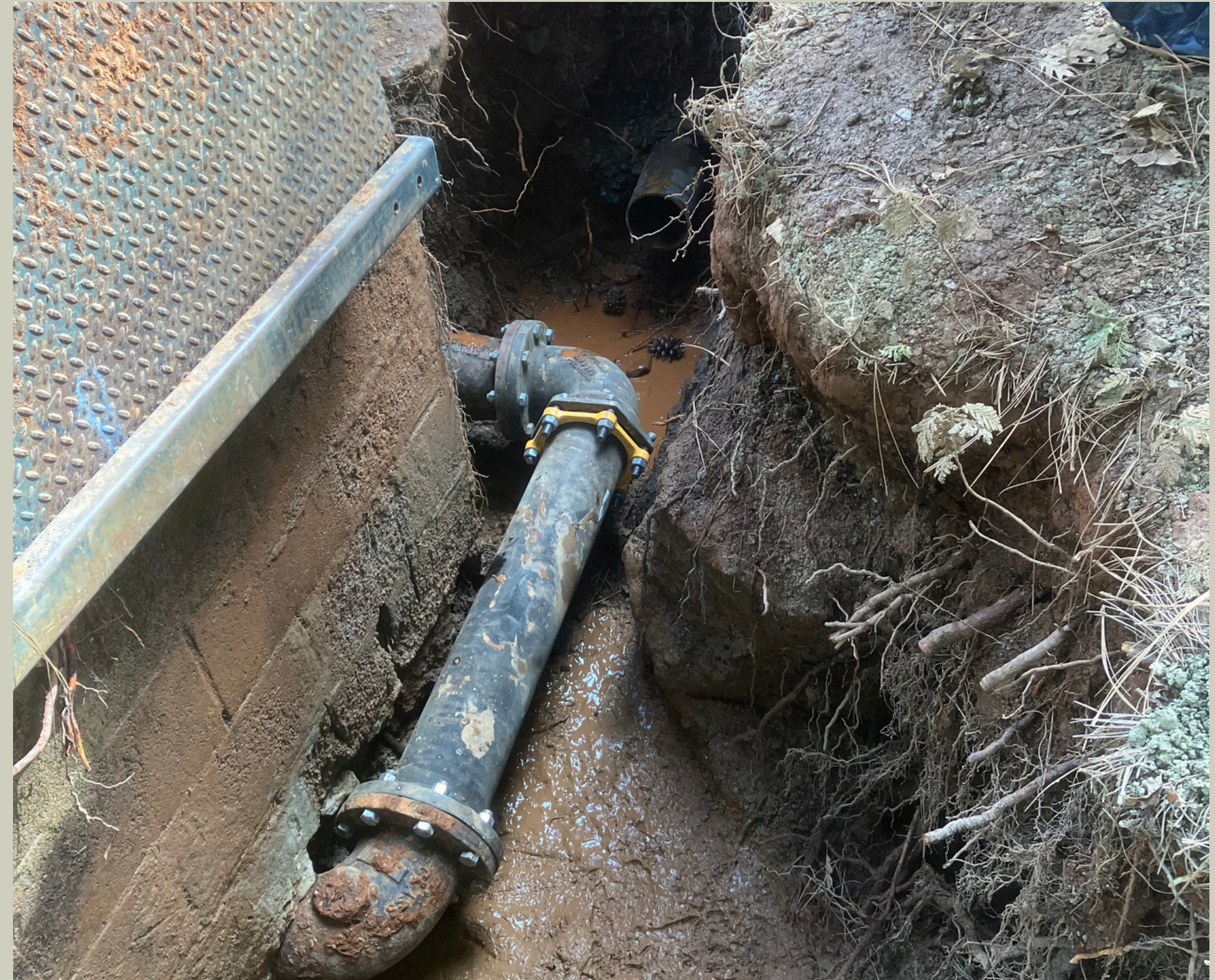
Leak at PRV 30 on Thunderbolt - Ebbetts Pass
