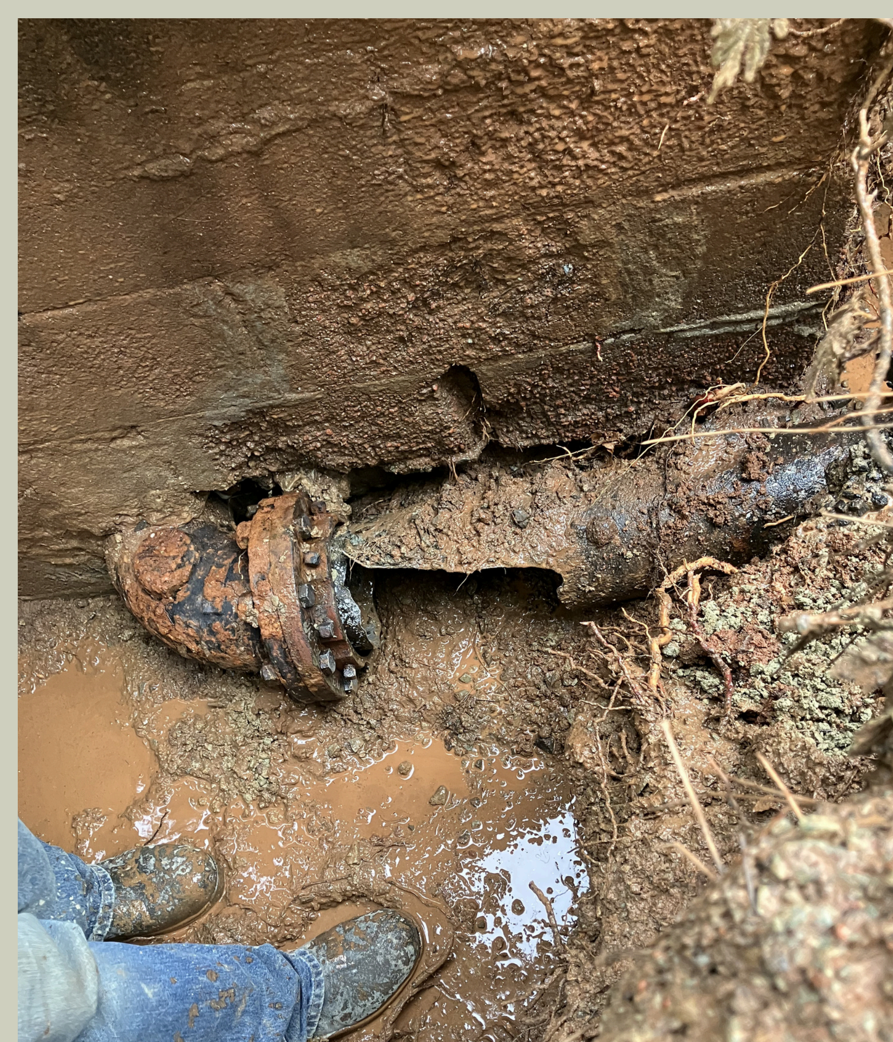
Leak at PRV 30 on Thunderbolt - Ebbetts Pass
