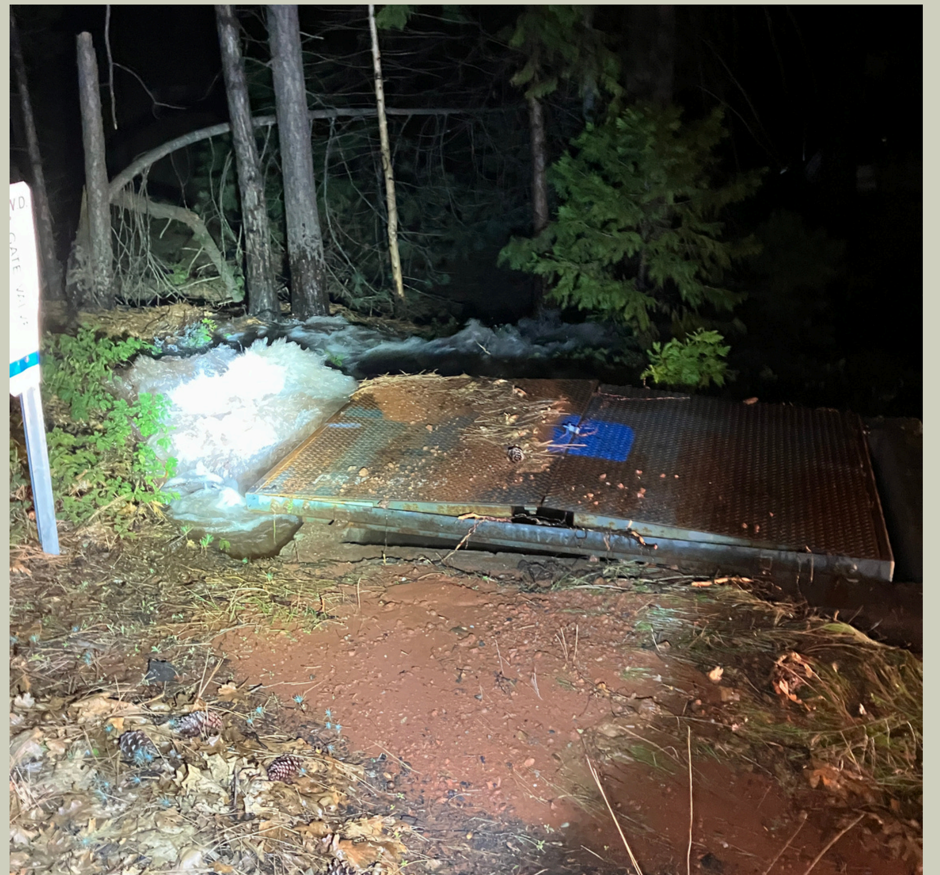
Leak at PRV 30 on Thunderbolt - Ebbetts Pass
