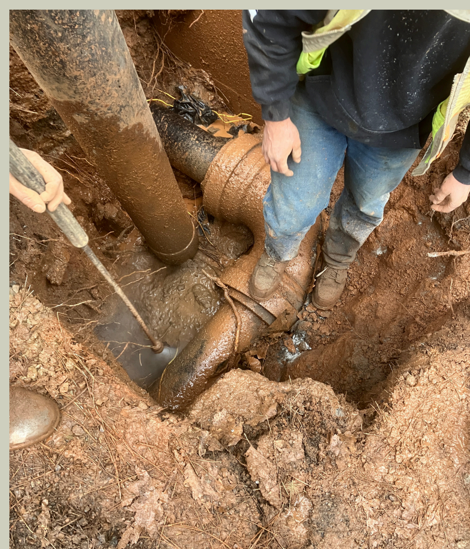
Leak at PRV 30 on Thunderbolt - Ebbetts Pass
