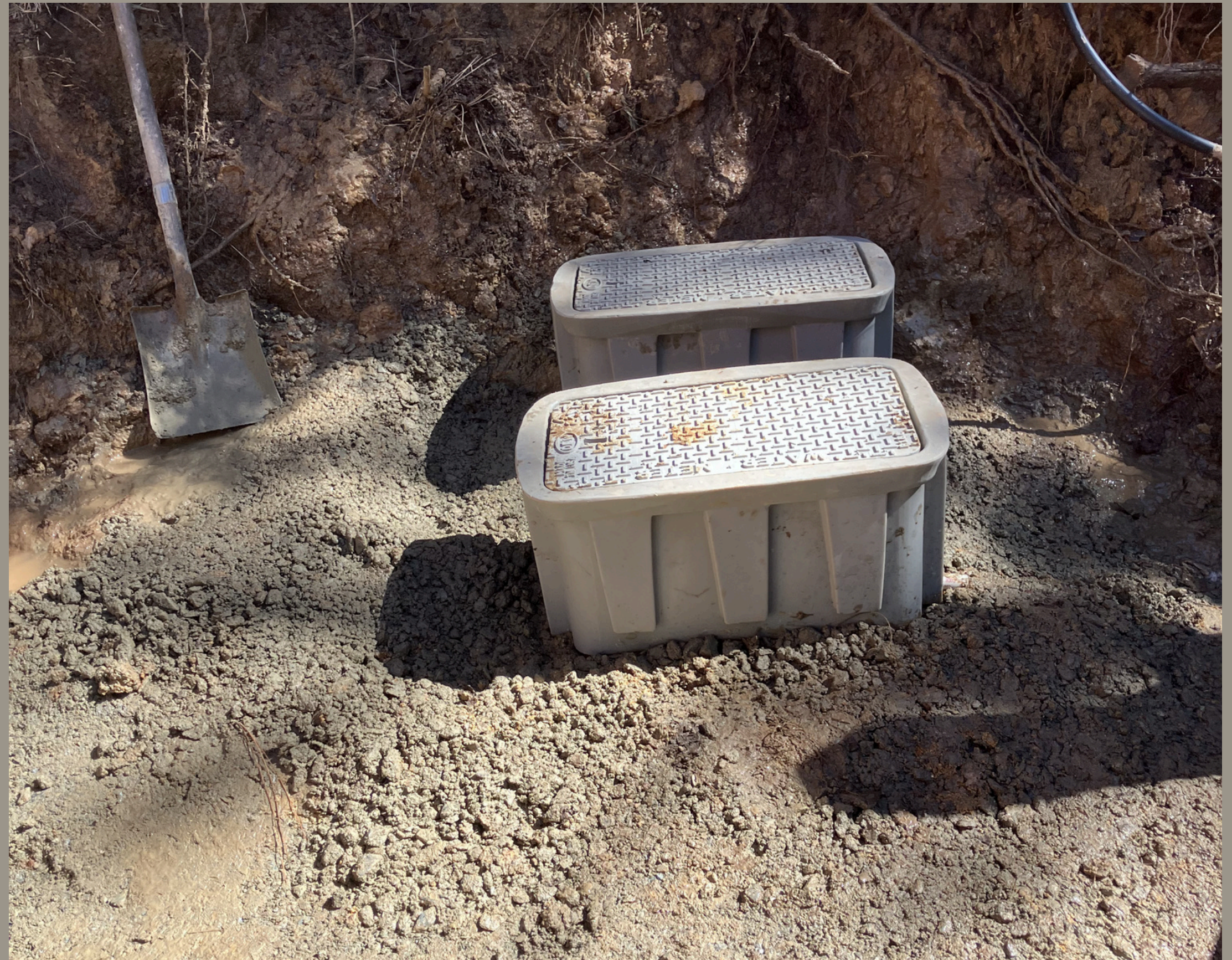
Lilac Drive Service Line Repair - Ebbetts Pass
