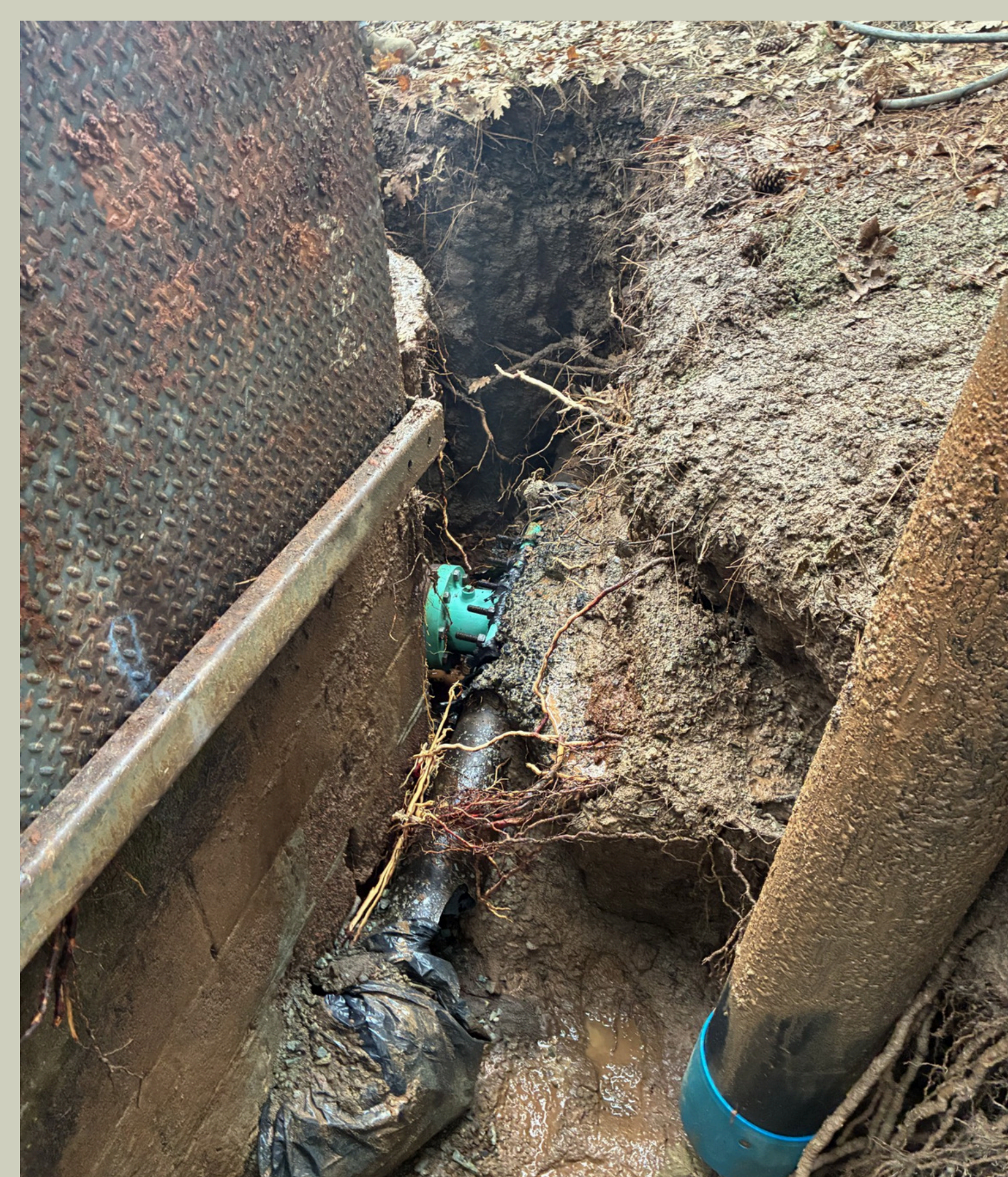
Leak at PRV 30 on Thunderbolt - Ebbetts Pass
