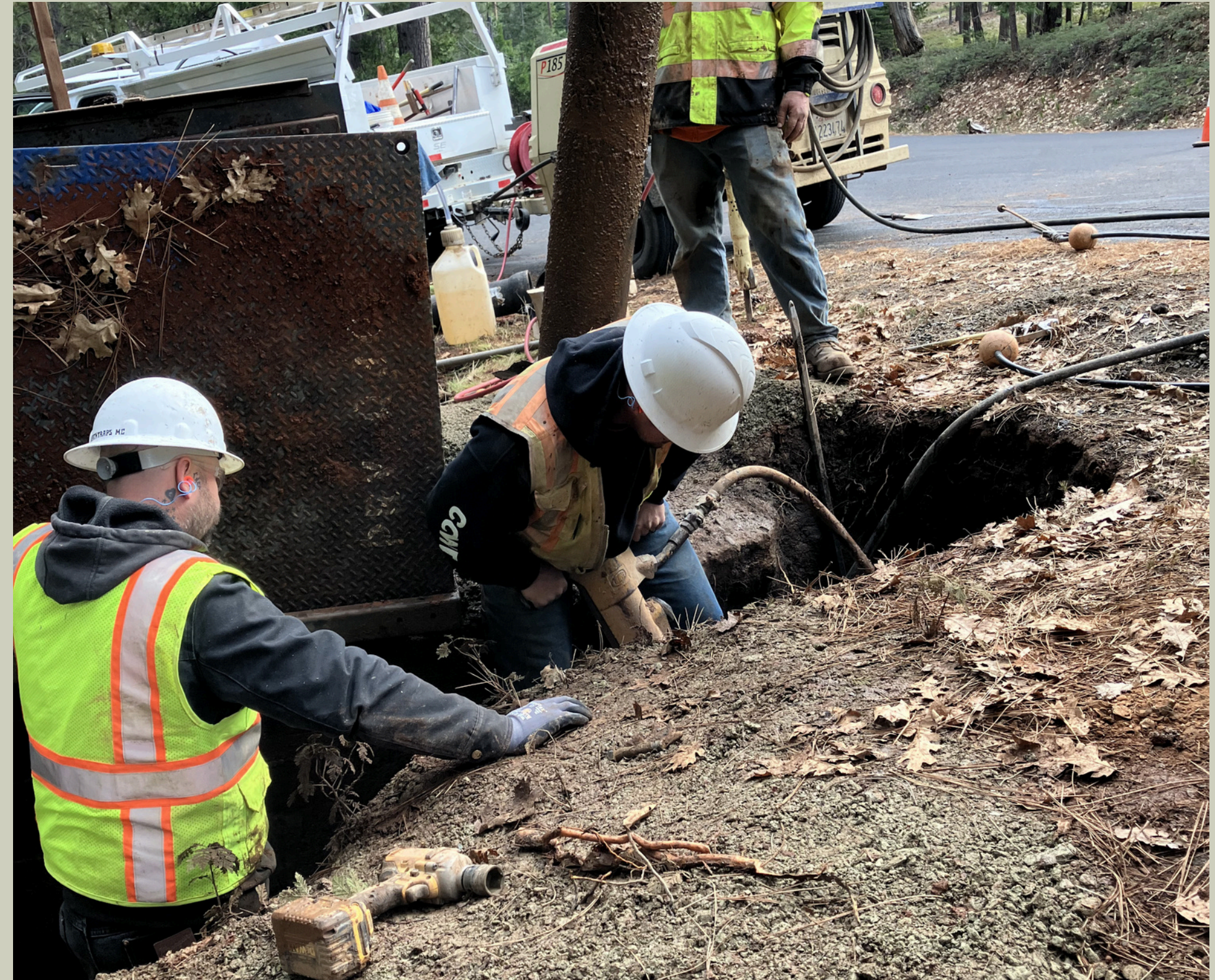
Leak at PRV 30 on Thunderbolt - Ebbetts Pass
