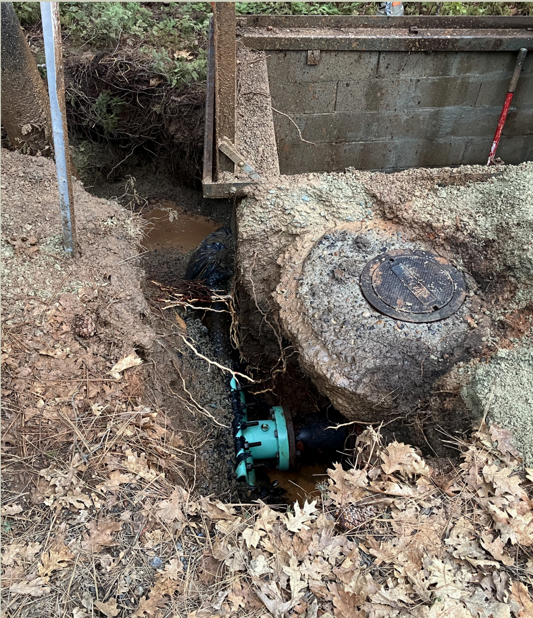
Leak at PRV 30 on Thunderbolt - Ebbetts Pass
