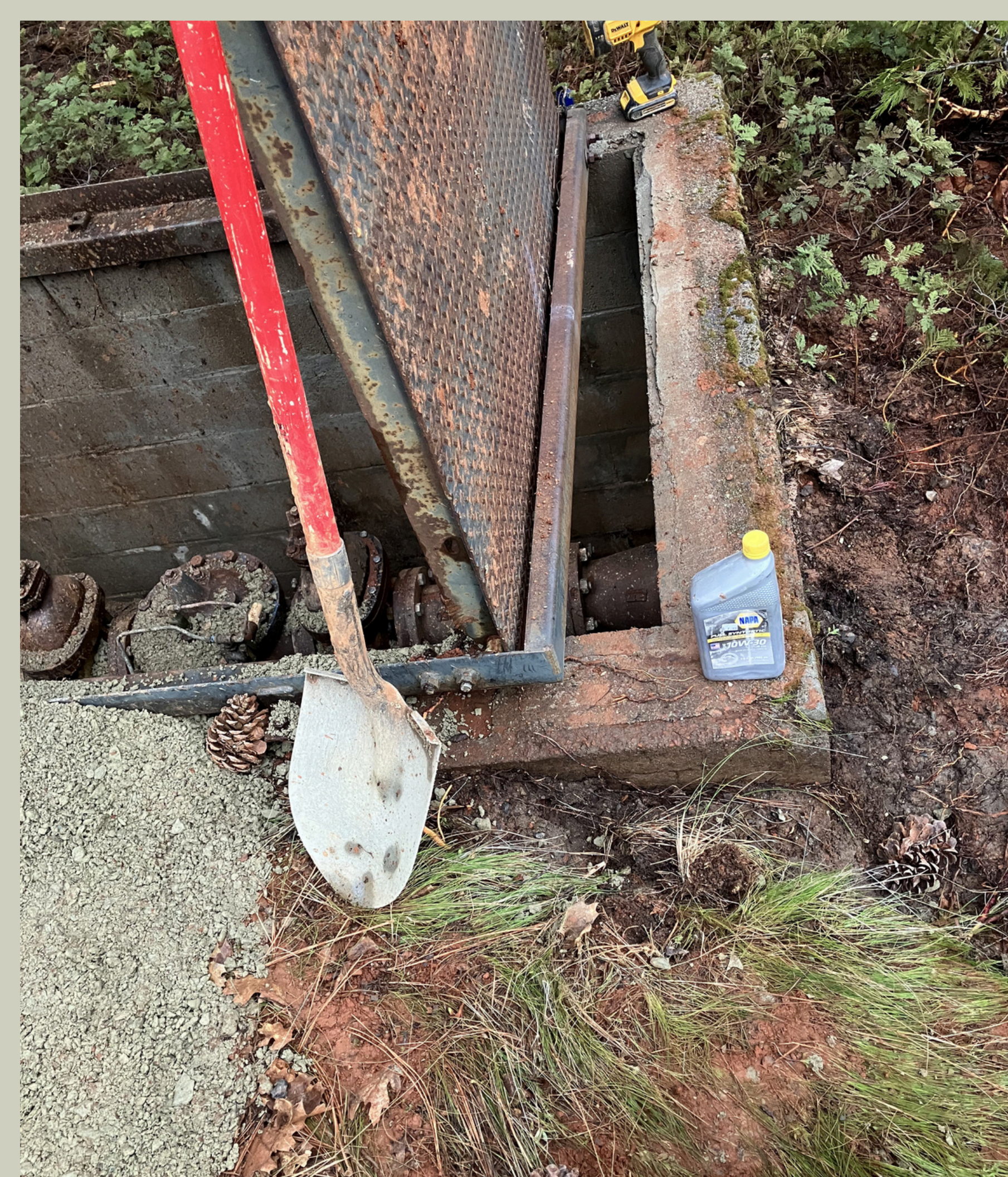
Leak at PRV 30 on Thunderbolt - Ebbetts Pass
