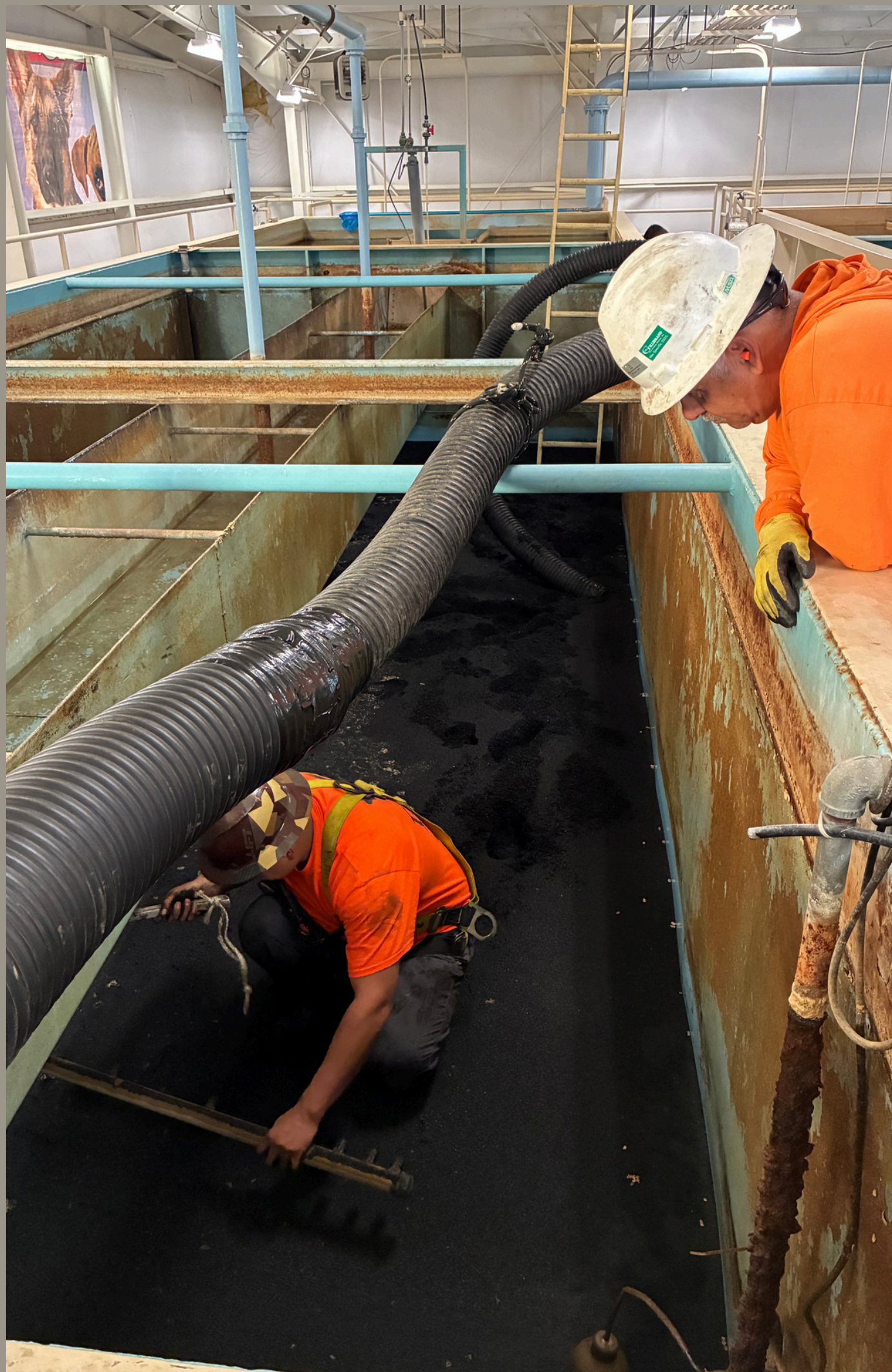
Began Filter Rehabilitation Project - Copper Cove WTP
