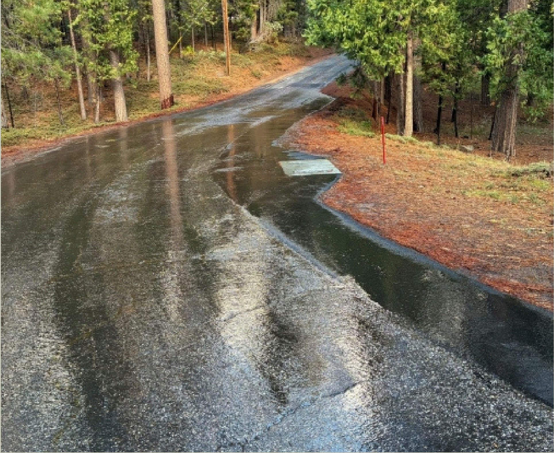
Leak at PRV 30 on Thunderbolt - Ebbetts Pass
