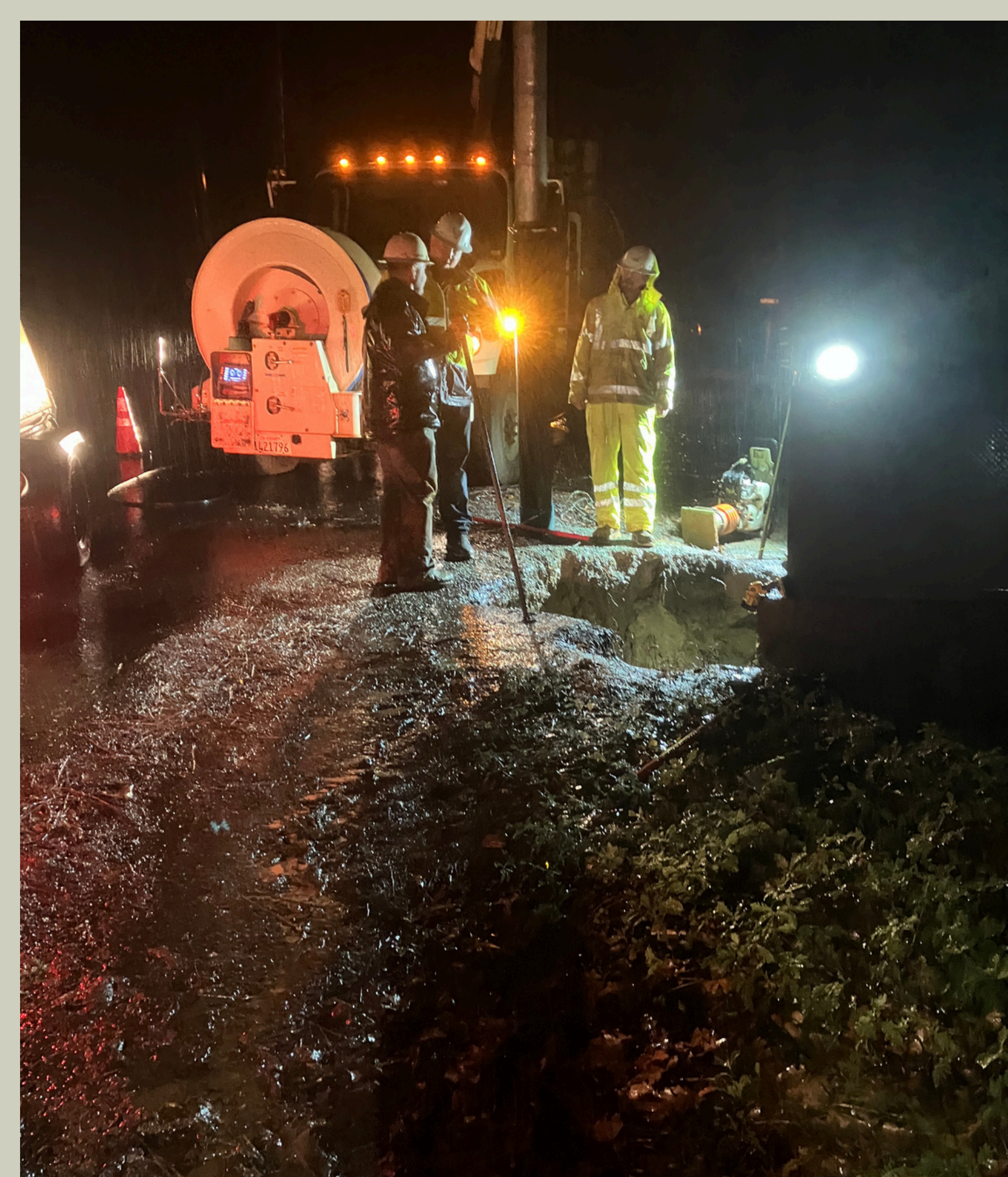
Leak at PRV 30 on Thunderbolt - Ebbetts Pass
