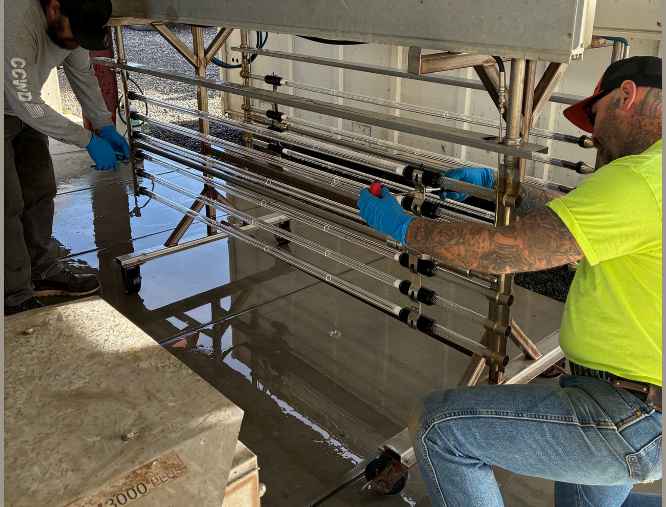
UV System Maintenance - Copper Cove Reclamation Plant
