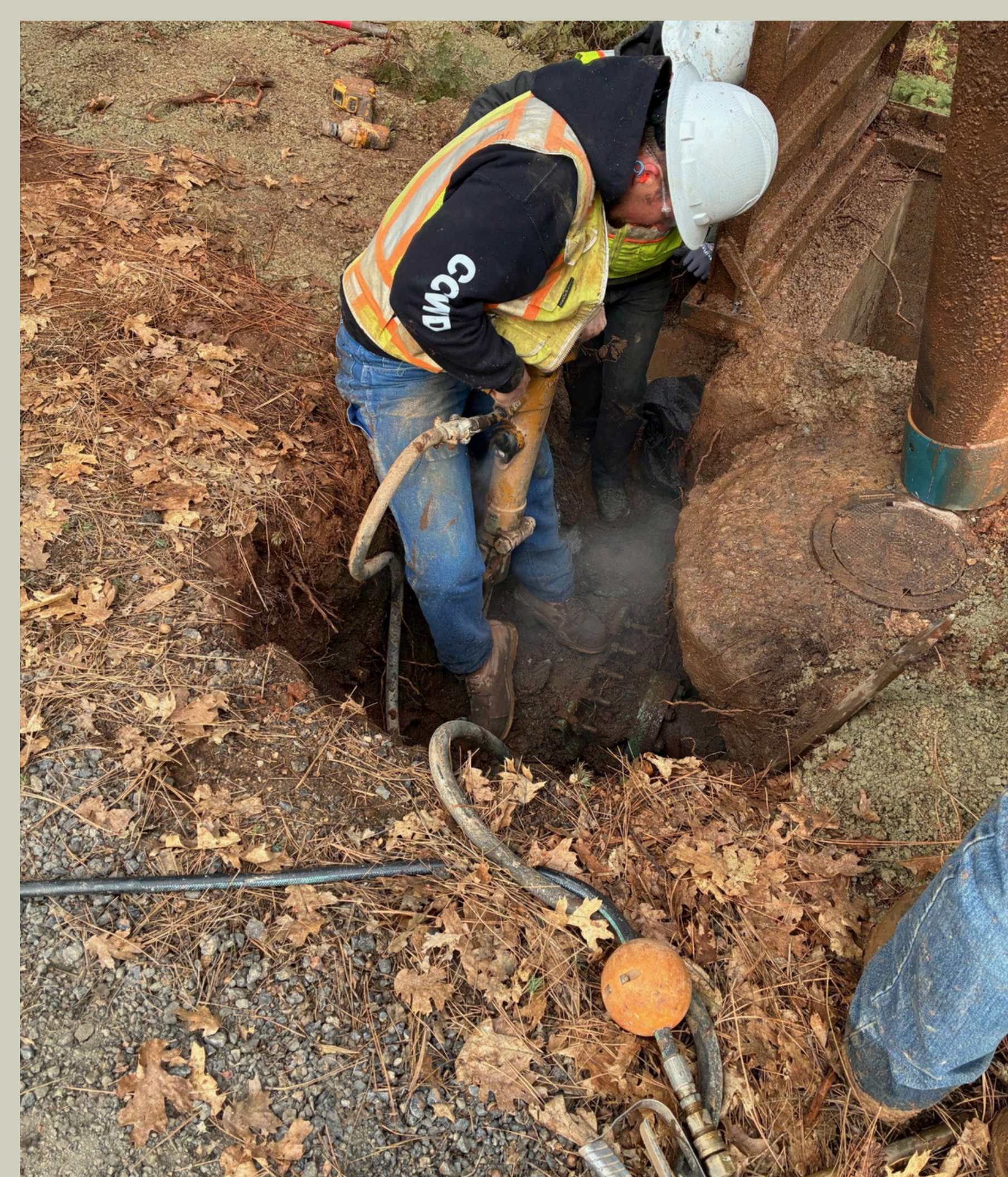
Leak at PRV 30 on Thunderbolt - Ebbetts Pass
