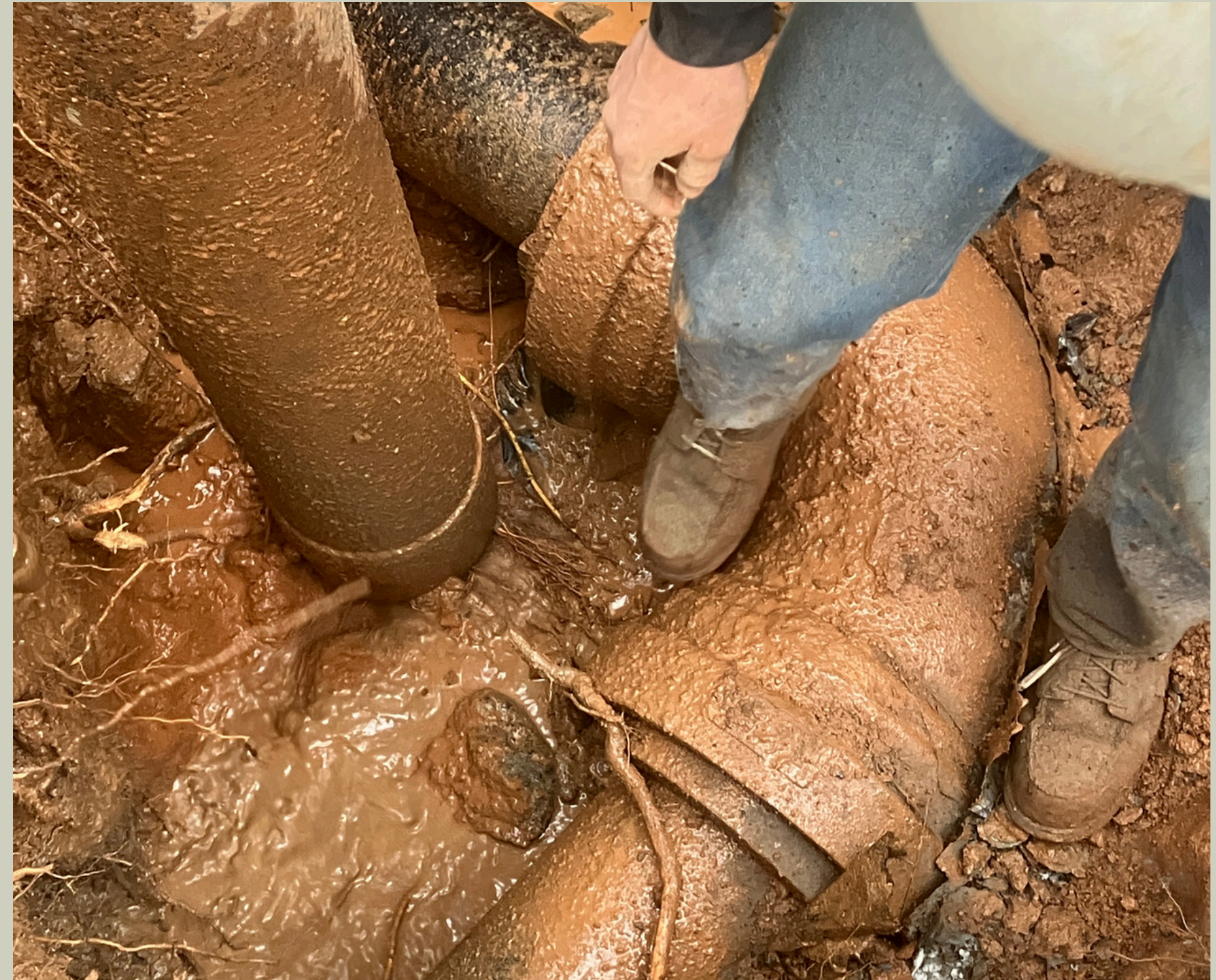
Leak at PRV 30 on Thunderbolt - Ebbetts Pass
