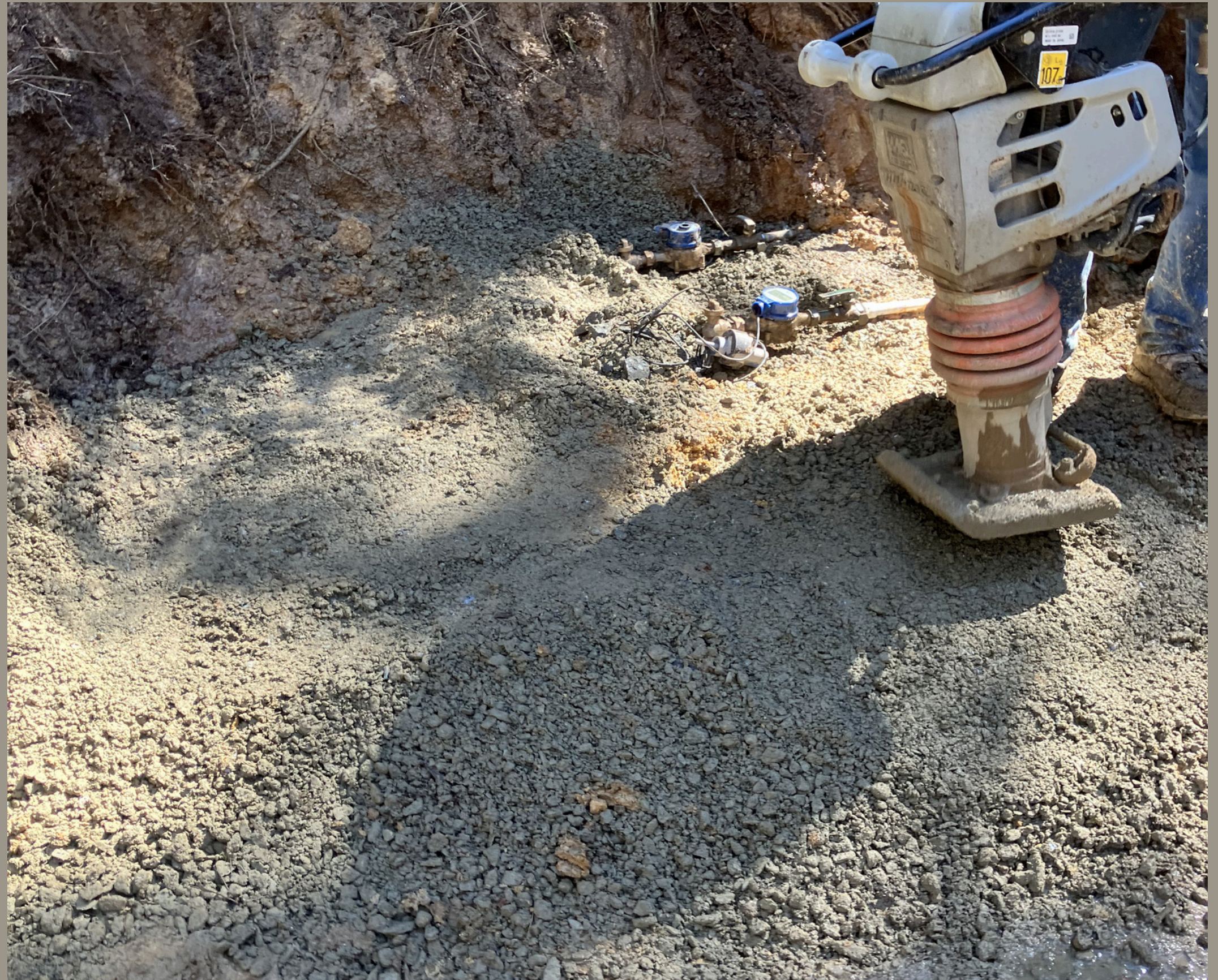
Lilac Drive Service Line Repair - Ebbetts Pass
