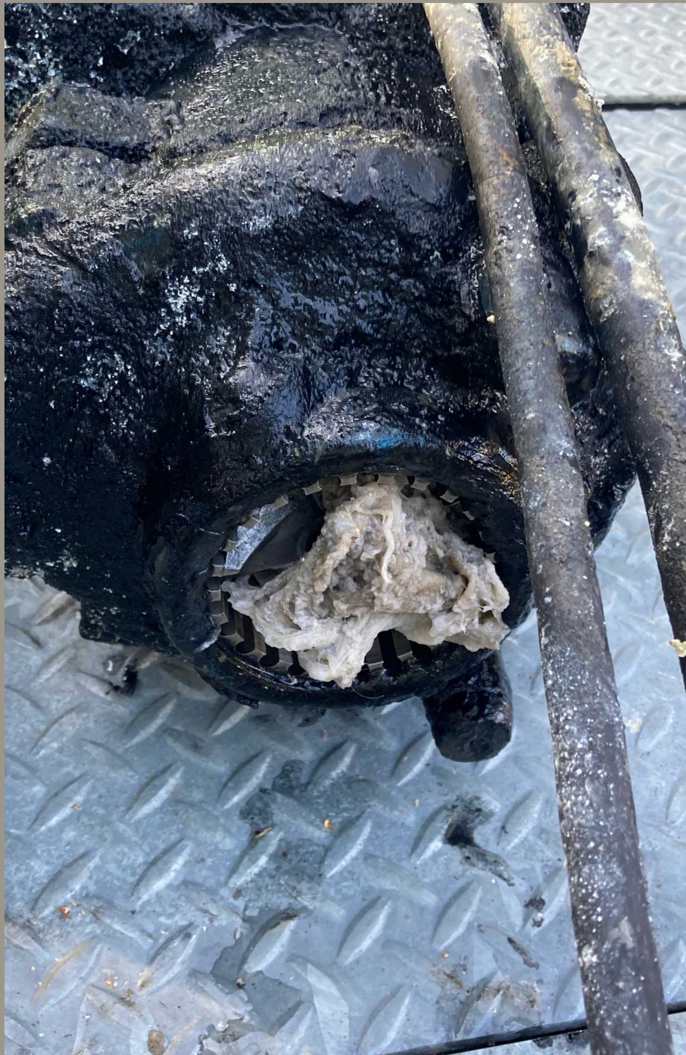
De-Ragged Pumps at Lift Station 10 - Poker Flat
