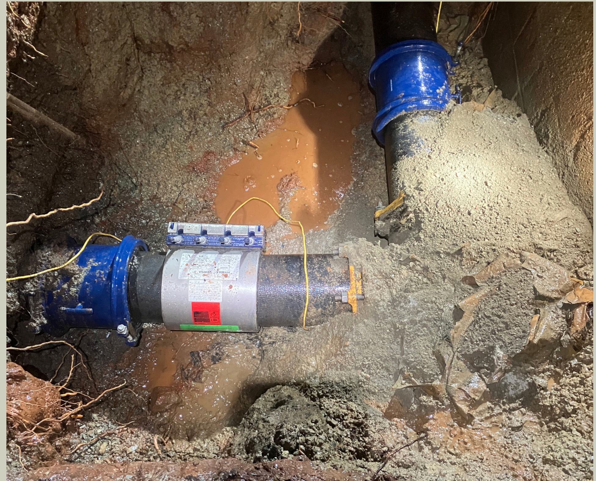
Leak at PRV 30 on Thunderbolt - Ebbetts Pass
