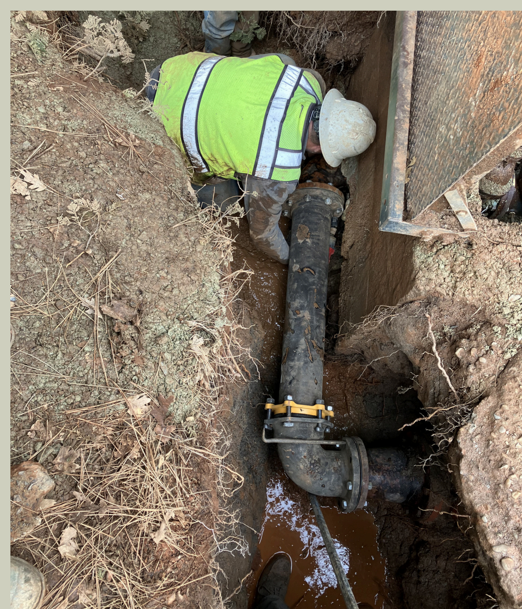
Leak at PRV 30 on Thunderbolt - Ebbetts Pass
