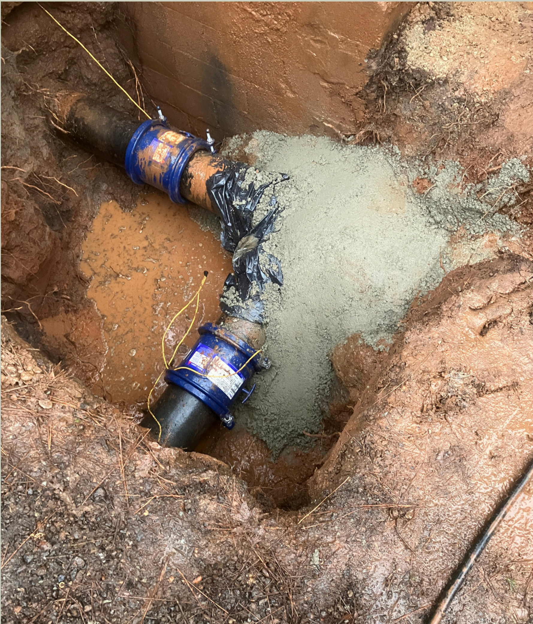
Leak at PRV 30 on Thunderbolt - Ebbetts Pass
