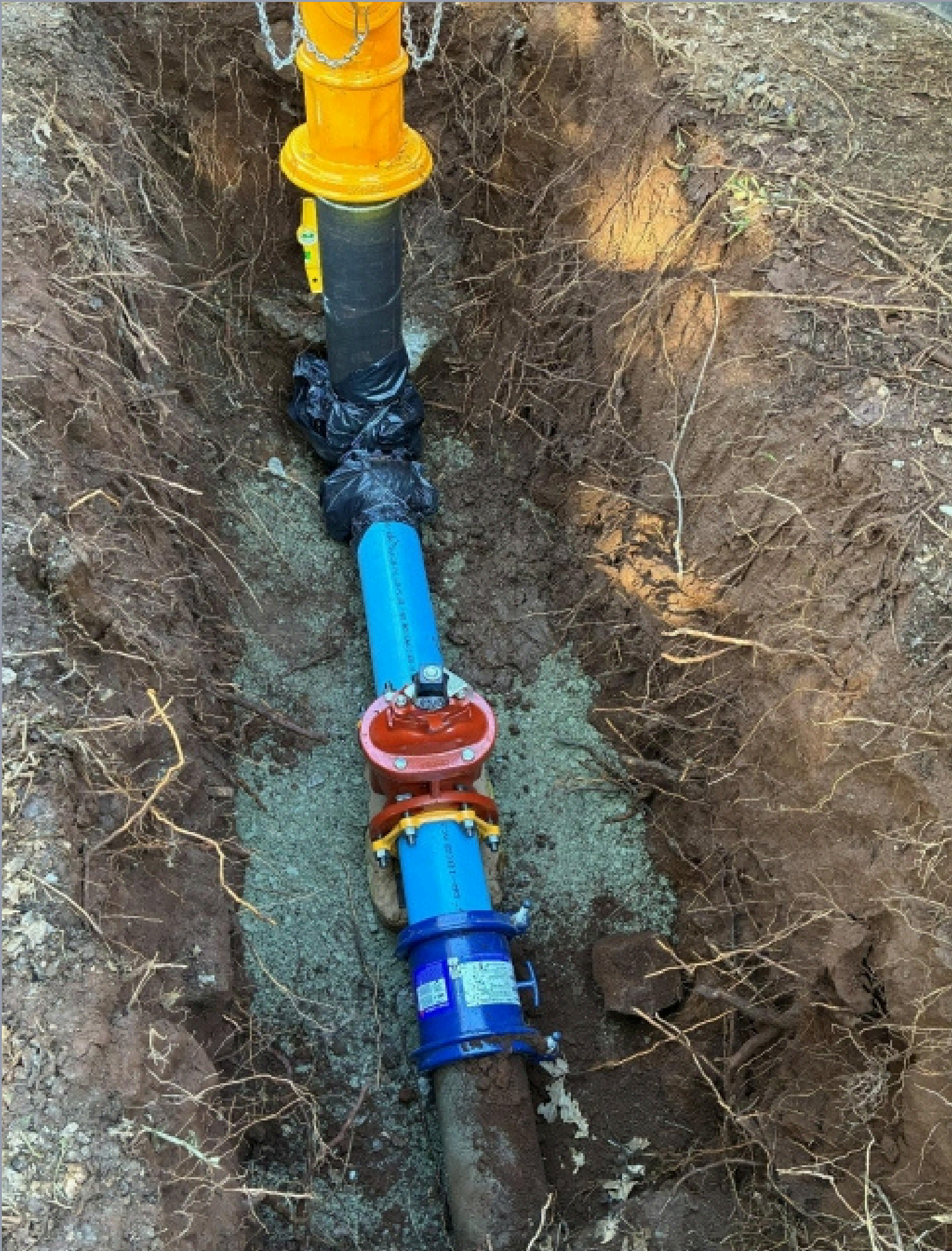
Fire Hydrant Replacement - Manual Road - Arnold
