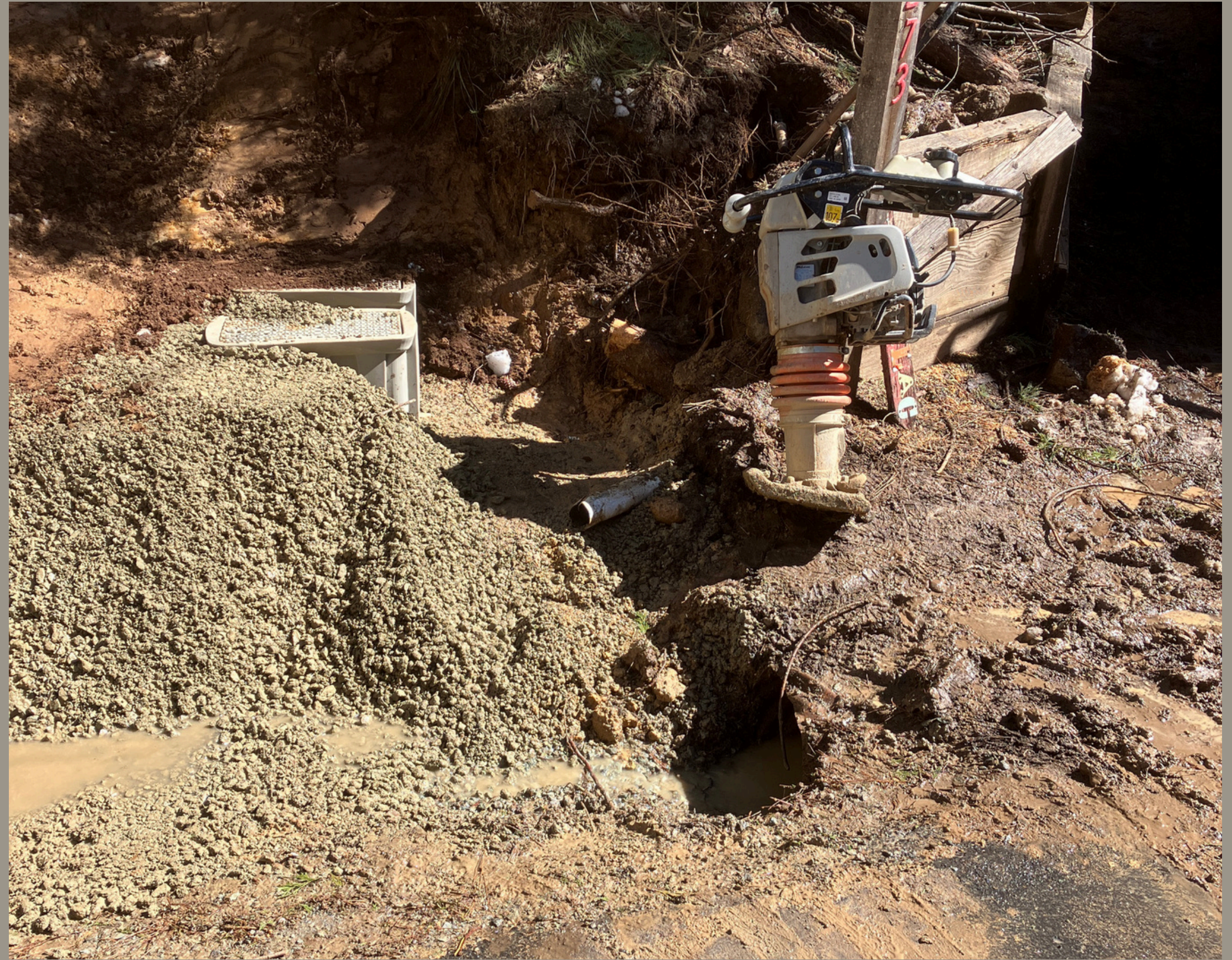
Lilac Drive Service Line Repair - Ebbetts Pass
