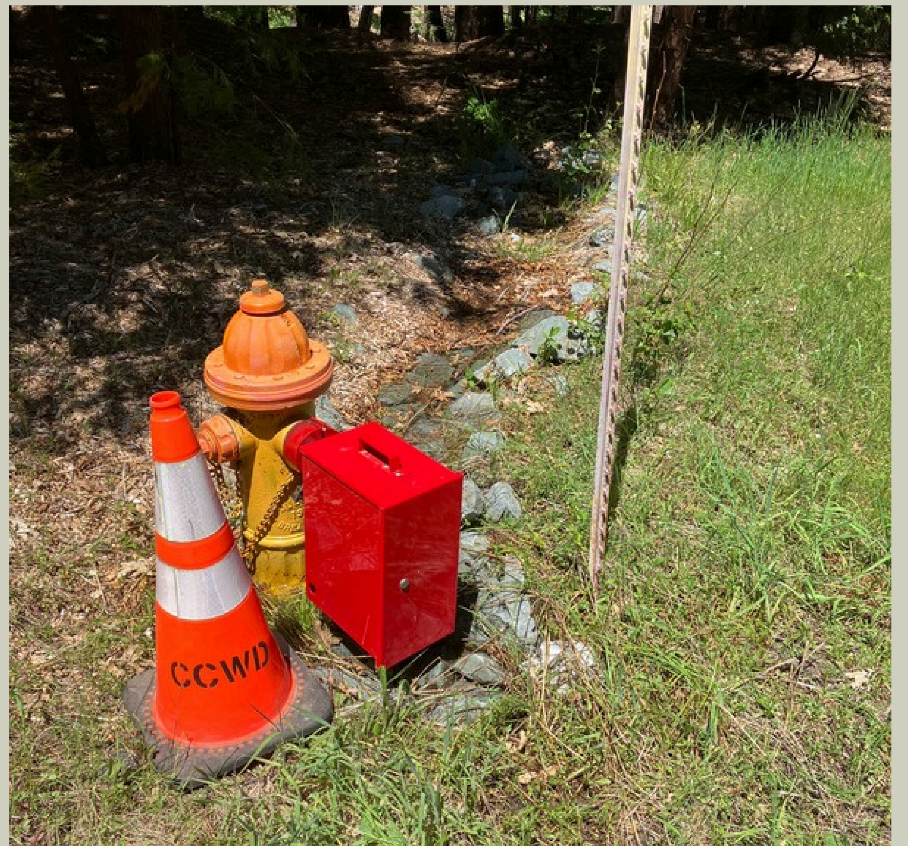
Autoflushers Deployed - Big Trees Village - Ebbetts Pass
