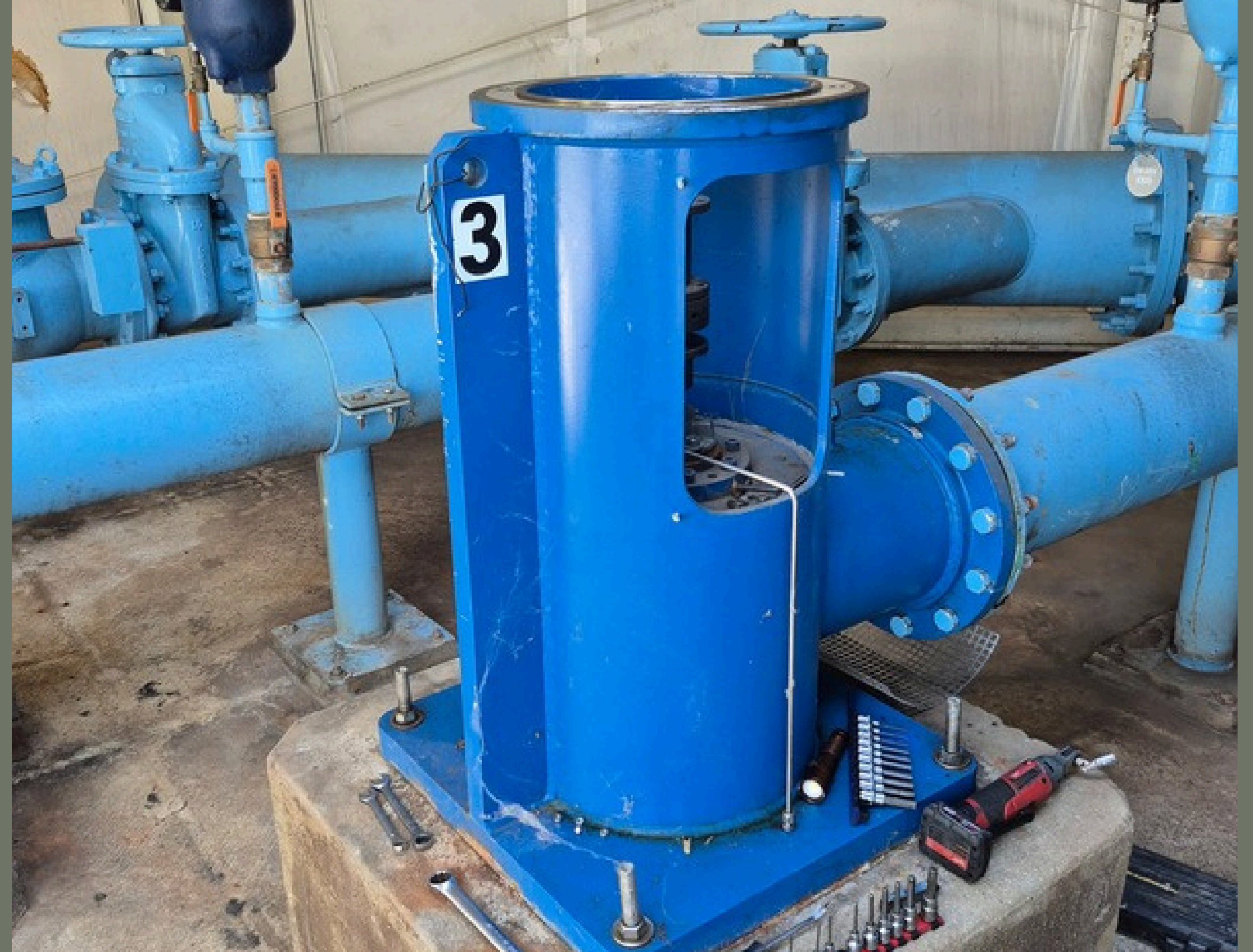
Electrical + Mechanical - Replacing Raw Pump 3 Motor - Jenny Lind WTP
