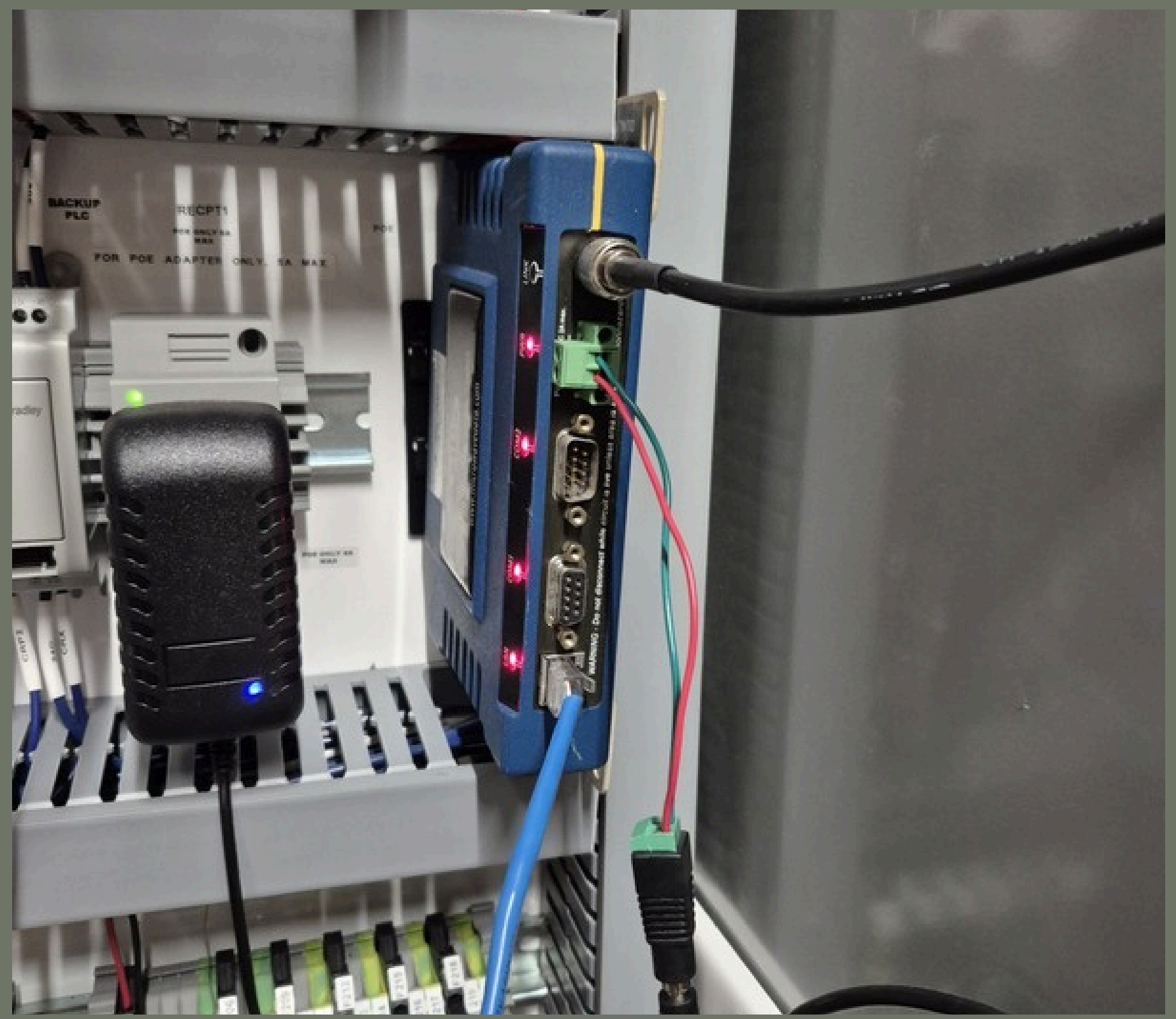
Electricians - Troubleshoot Comm Fail - Wilseyville Lift Station
