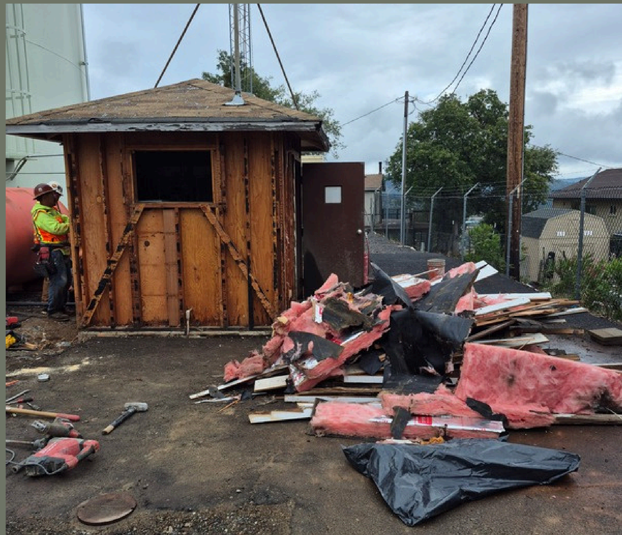
Electrical - Prepping the C Tank Hydro BLDG For Rehab - Copper
