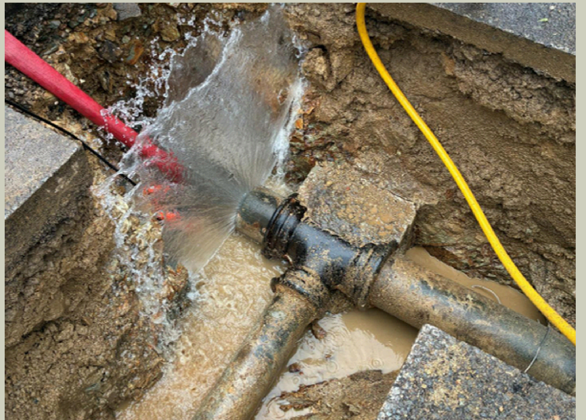
8-inch, 6-inch valve replacement and water line abandonment - Hartvickson - Rancho Calaveras
