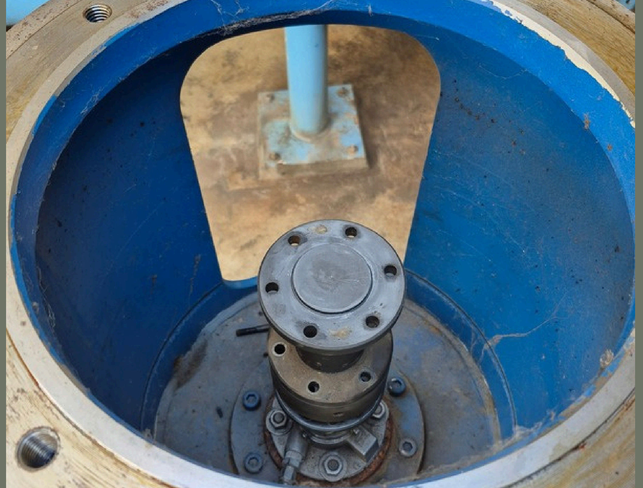
Electrical + Mechanical - Replacing Raw Pump 3 Motor - Jenny Lind WTP
