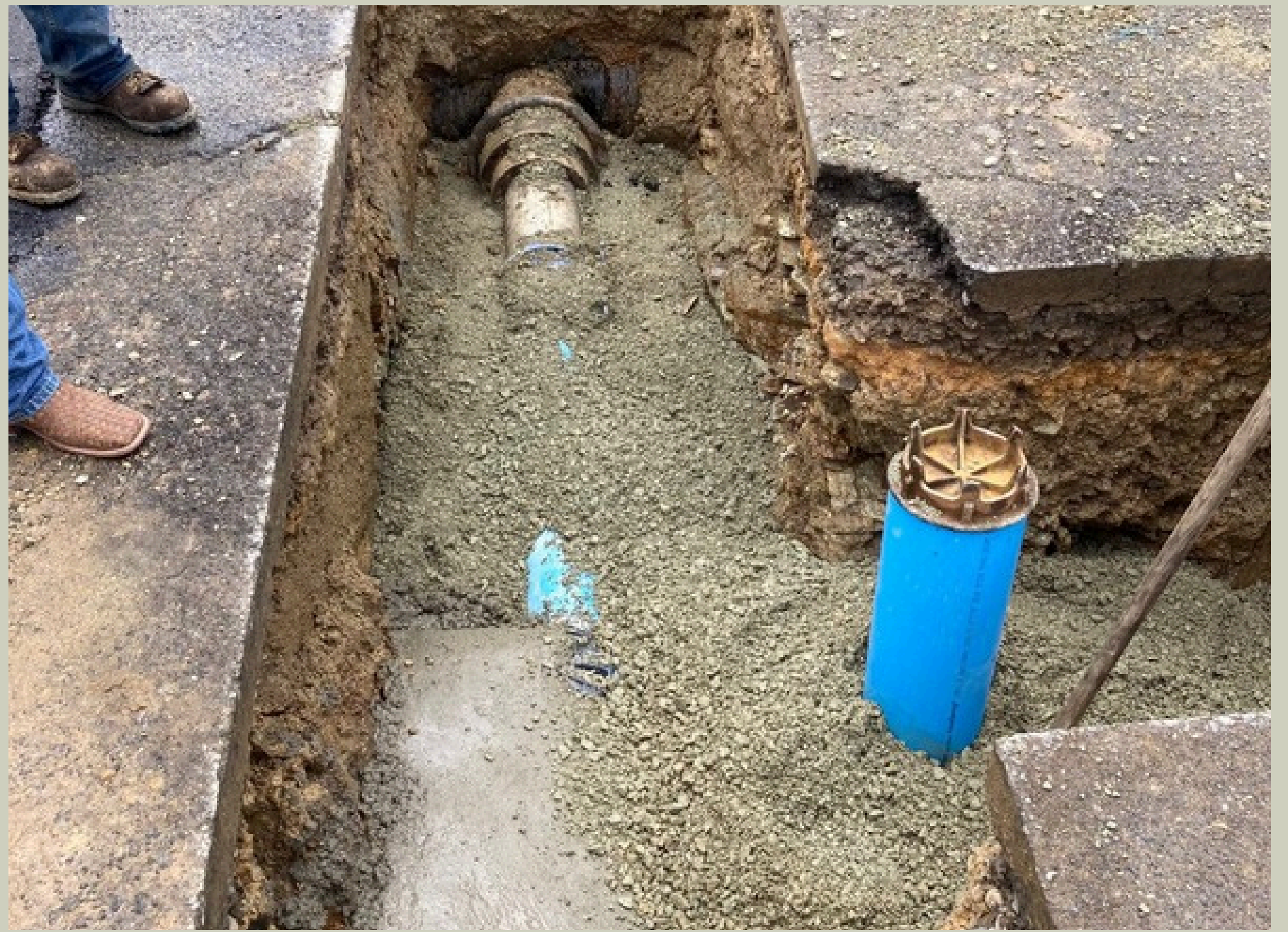
8-inch, 6-inch valve replacement and water line abandonment - Hartvickson - Rancho Calaveras
