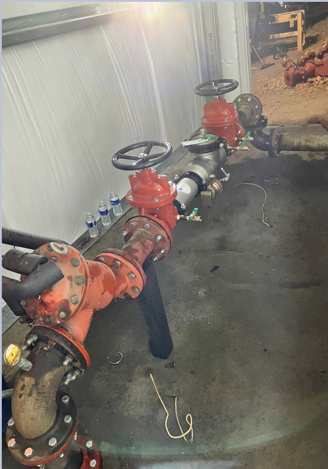
RP Backflow Prevention Device - Replacement - Big Trees Shopping Center
