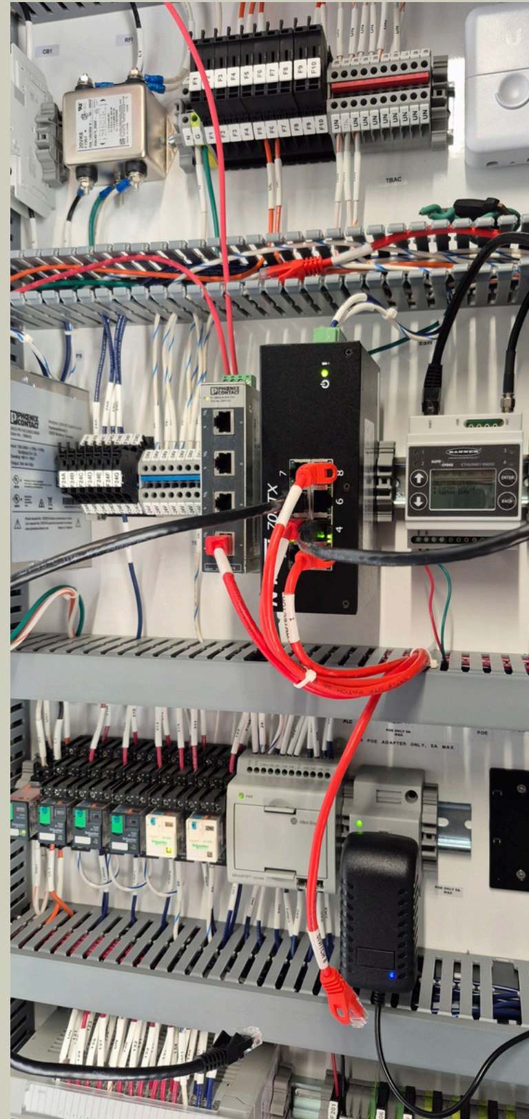
Electrical - Troubleshoot the Radio and HMI Conflict - Wilseyville Lift Station
