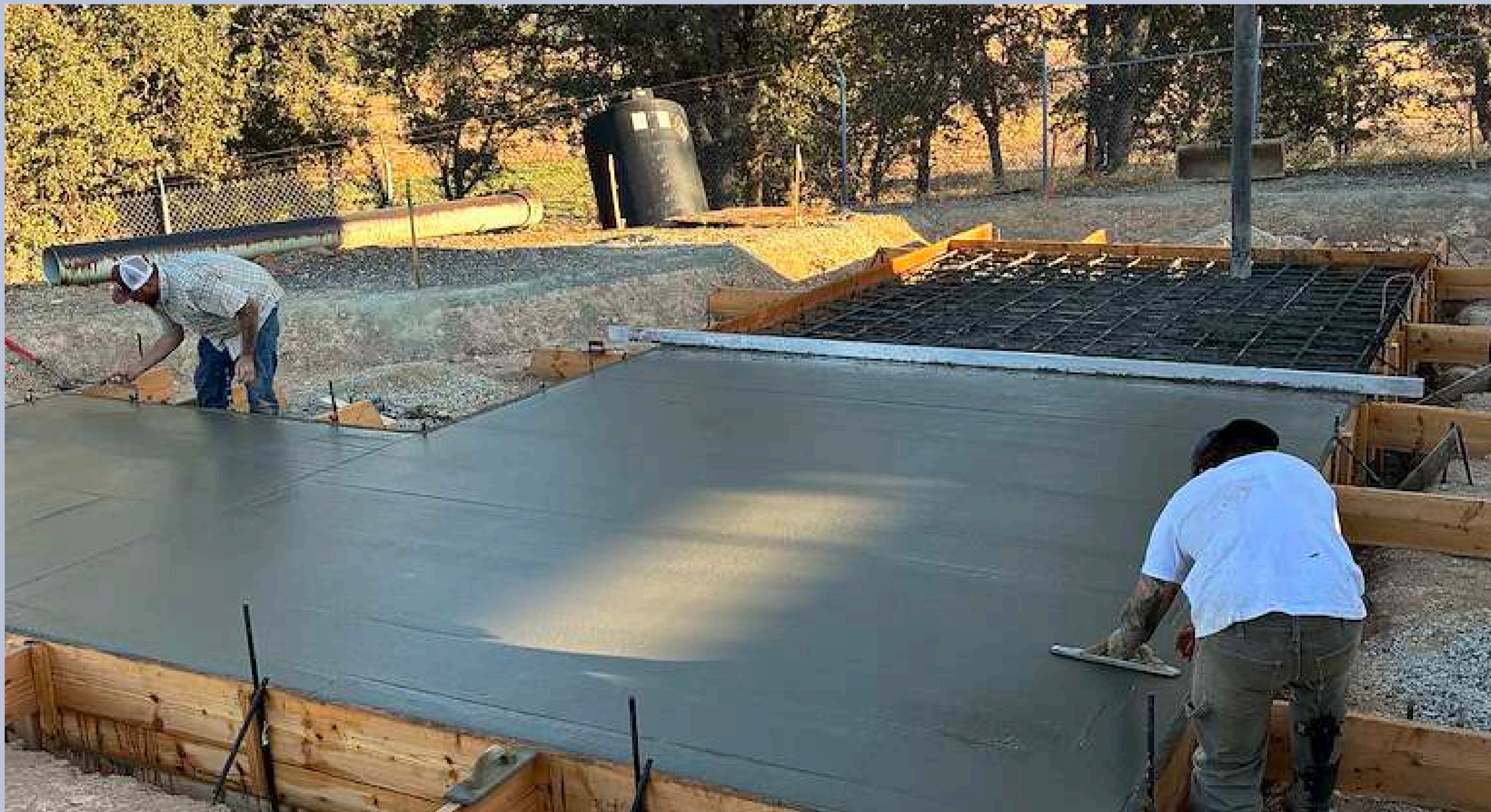
Construction - Site work and Pad Construction - SAF pre-treatment unit - Copper Reclaim
