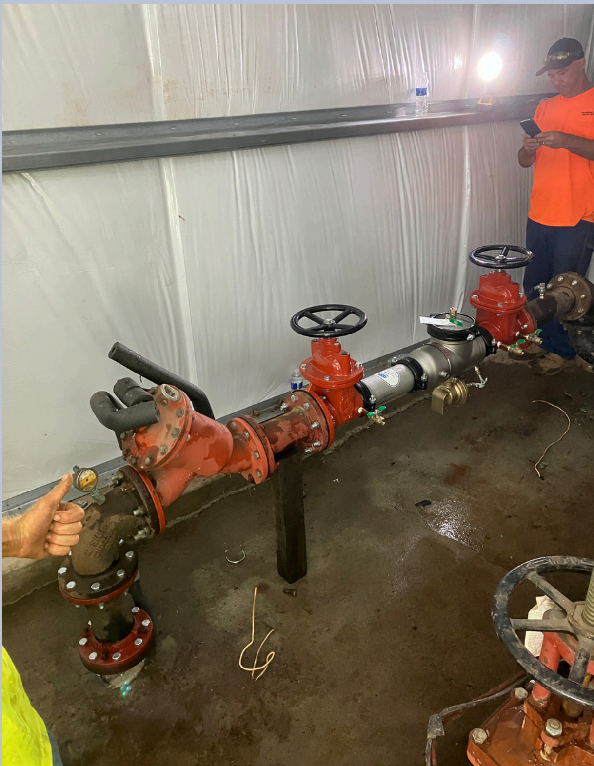
RP Backflow Prevention Device - Replacement - Big Trees Shopping Center
