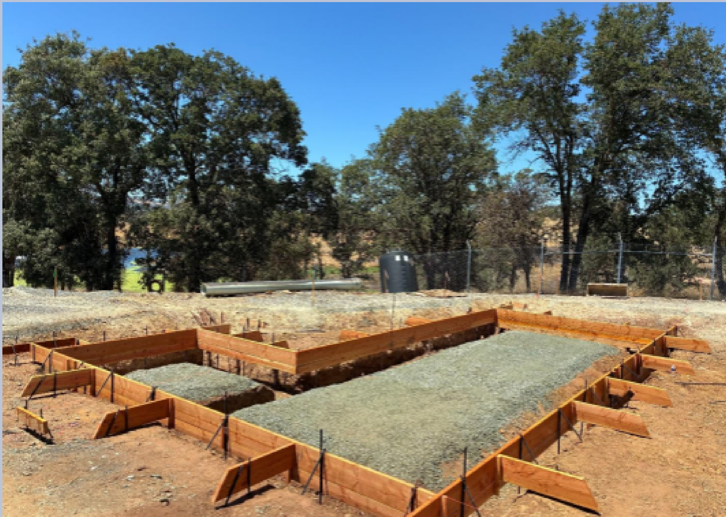
Construction - Site work and Pad Construction - SAF pre-treatment unit - Copper Reclaim
