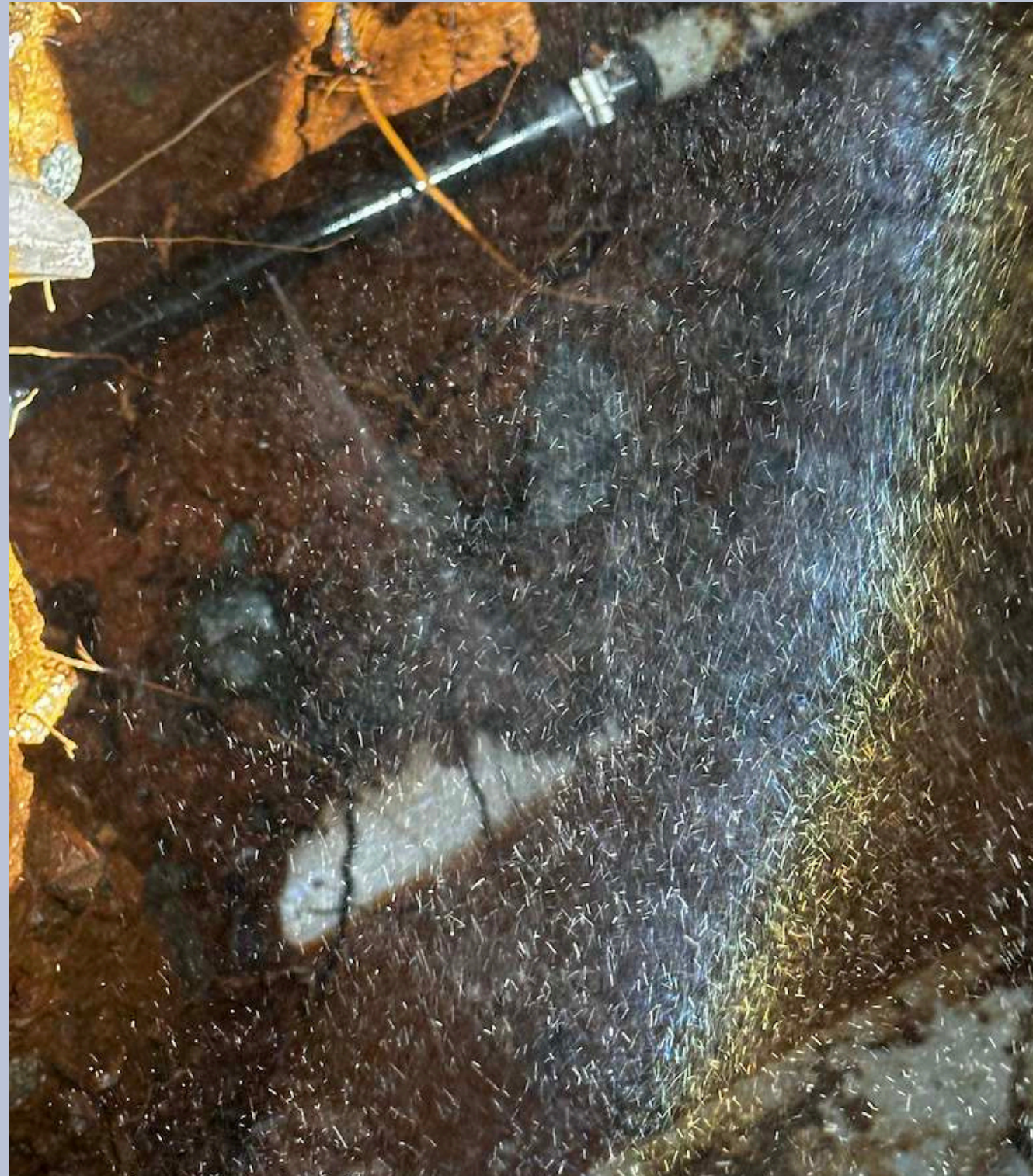
1 1/4 inch line Repair - Acorn - West Point
