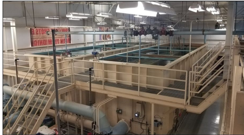
Copper Cove Water Treatment Plant
